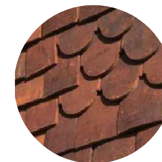
Upper Walls - Tile hanging
