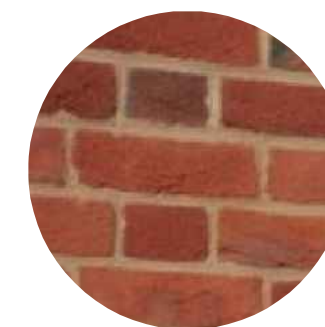
Lower Walls - Brick
