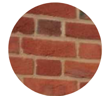
Lower Walls - Brick
