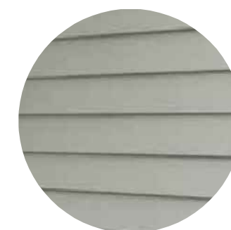
Upper Walls - Weatherboarding
