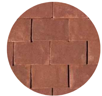
Roof - Clay tile
