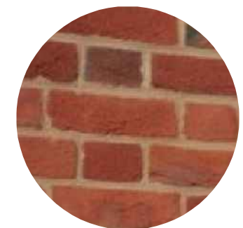
Lower Walls - Brick
