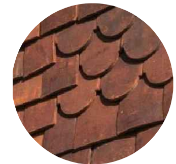
Upper Walls - Tile hanging
