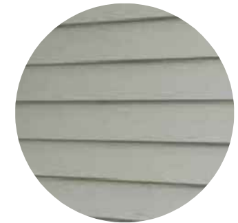
Upper Walls - Weatherboarding
