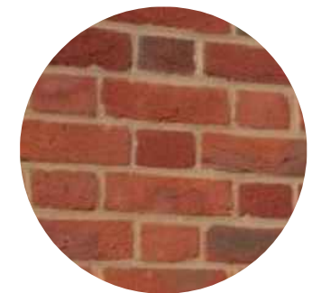
Lower Walls - Brickwork
