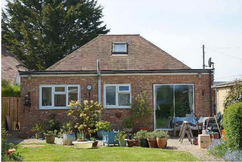
Fig.1: View looking to the rear of Alafin showing the flat roof area which is to be extended into the back garden. The existing roof will be replaced and the fletton brickwork will be vertically clad to match in with the proposal. The width of the new extension will be the same as the existing.
