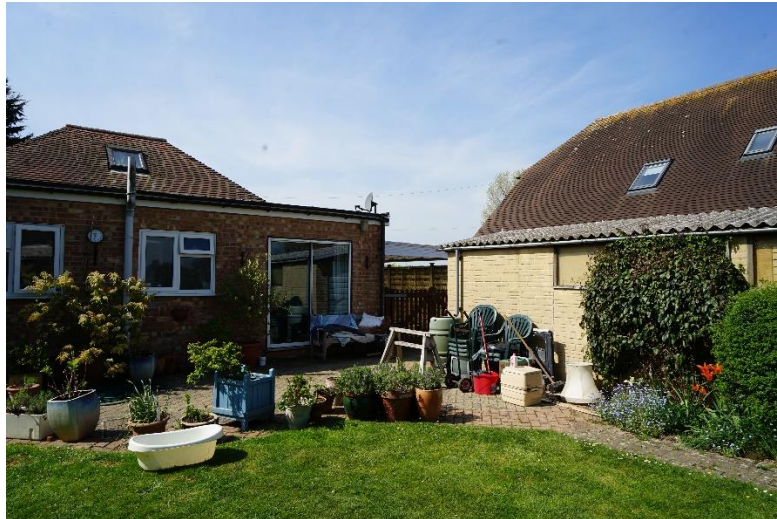
Fig.3: Part view of the rear of Alafin and the existing garage with the roof of neighbouring property, Hillcrest, in the background.
