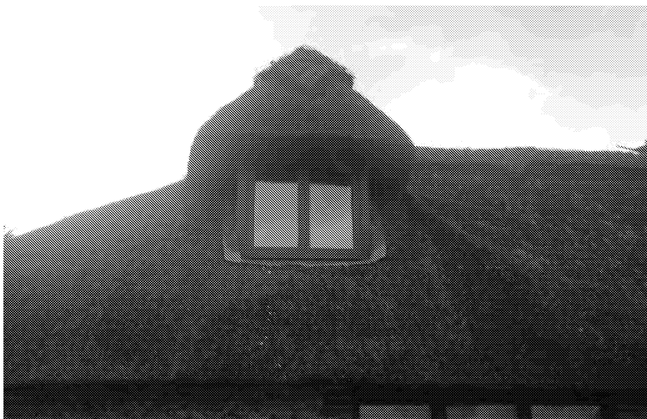
Appendix 4.4: Dormer window to the north east elevation of the Barn
