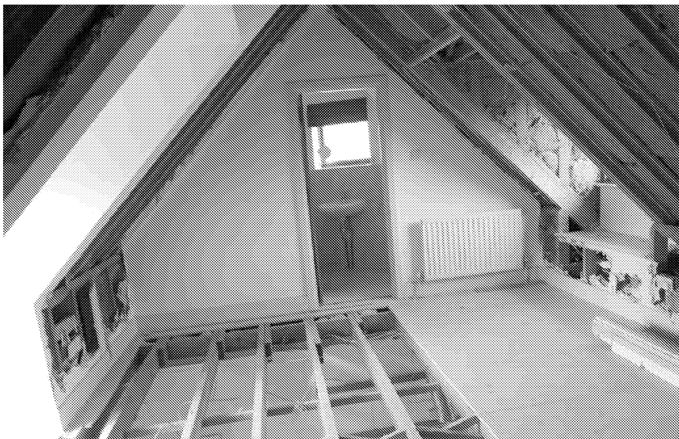
Appendix 4.14: First floor level of the late 20th century north addition to the Barn
