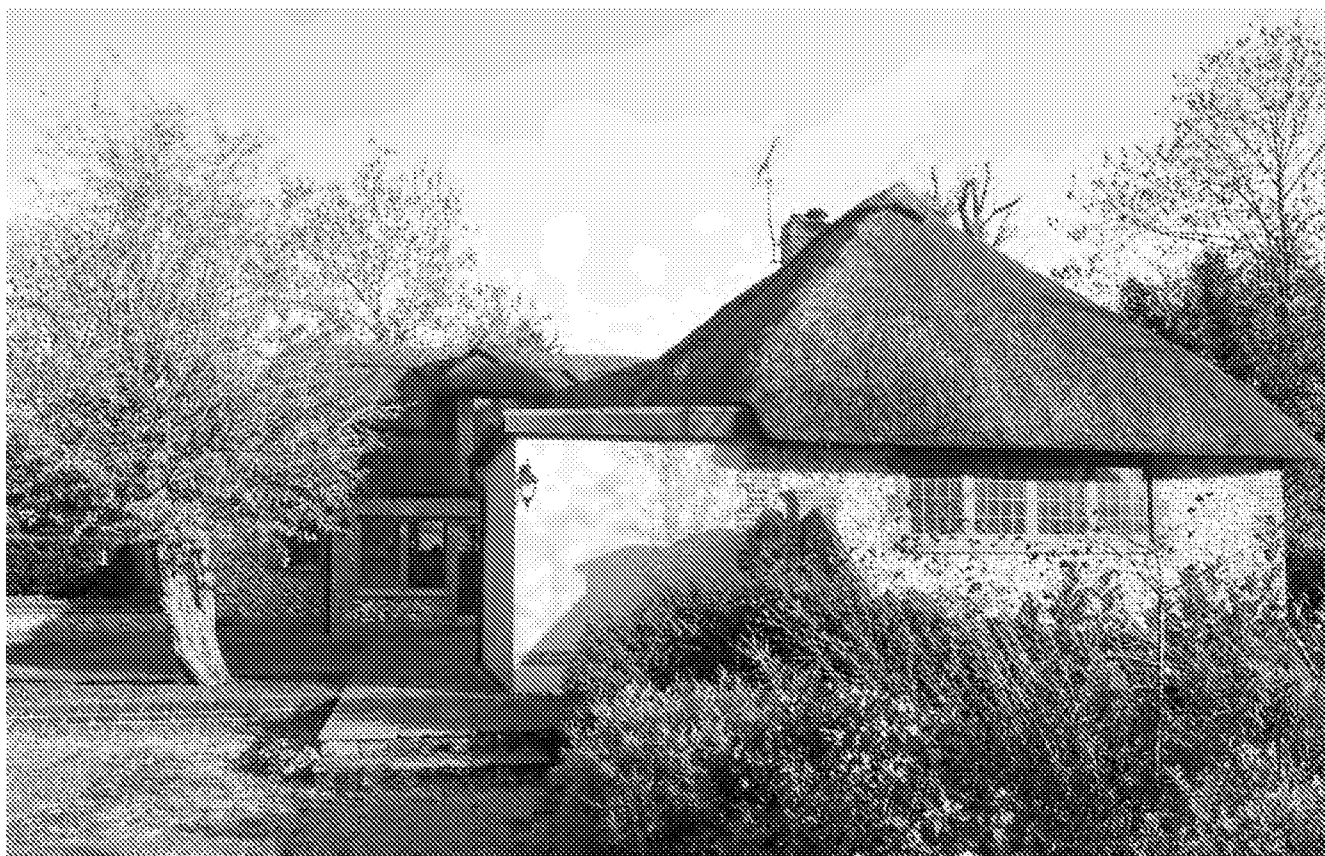
Appendix 4.5: South west elevation of the Barn
