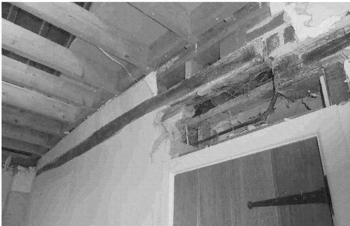
Appendix 4.15: Typical example of remnant timber framing found within the Barn
