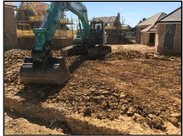
Plate 4: Back of excavator bucket lightly firming up the subsoil post ripping.
