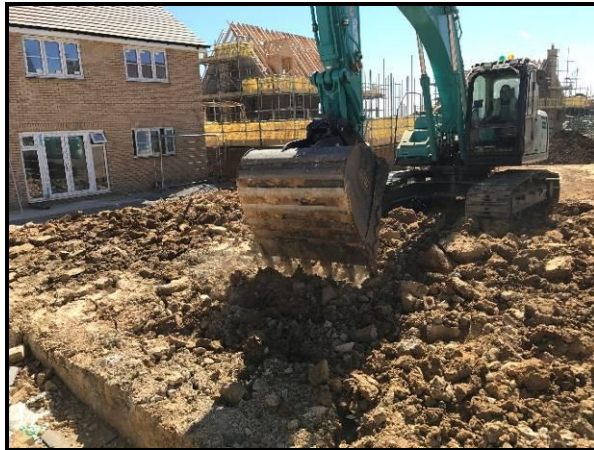
Plate 3: Toothed bucket breaking up large subsoil clods.
