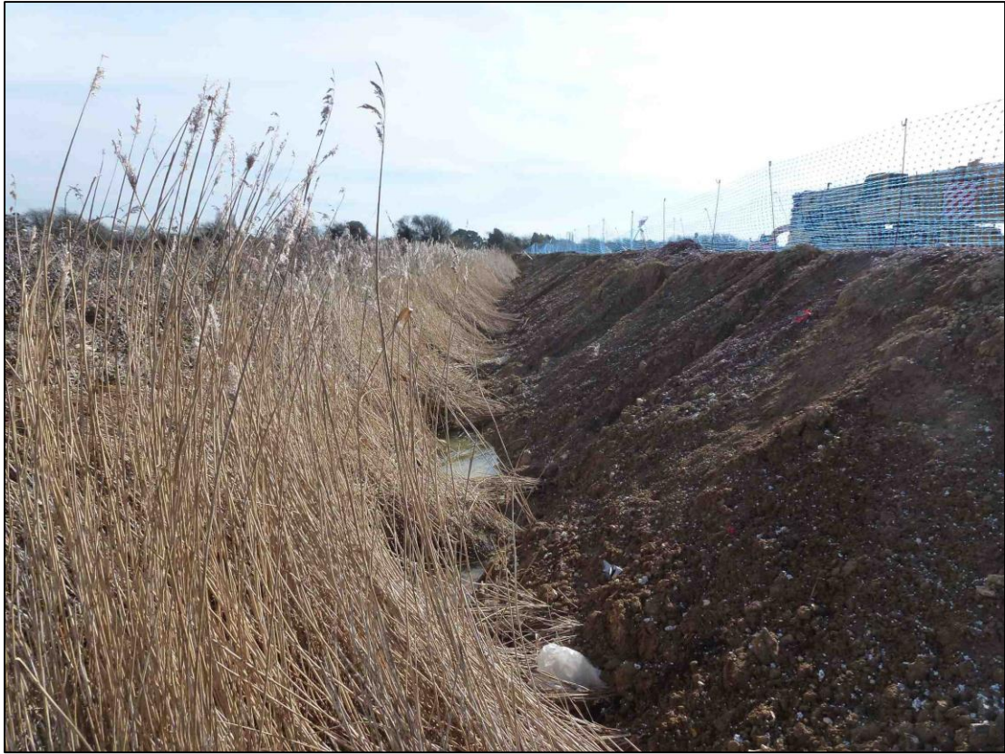
Photo 2: Watercourse along B2. The site is the left hand side of the ditch. The earth works on the right relate to the construction area of the new Roll Royce development.
