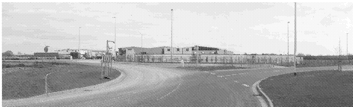
Rowan Way/A29 Shripney Road roundabout looking northeast towards the Oldlands Farm site entrance
