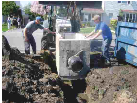
Smaller Smart Filter® being lowered into position
