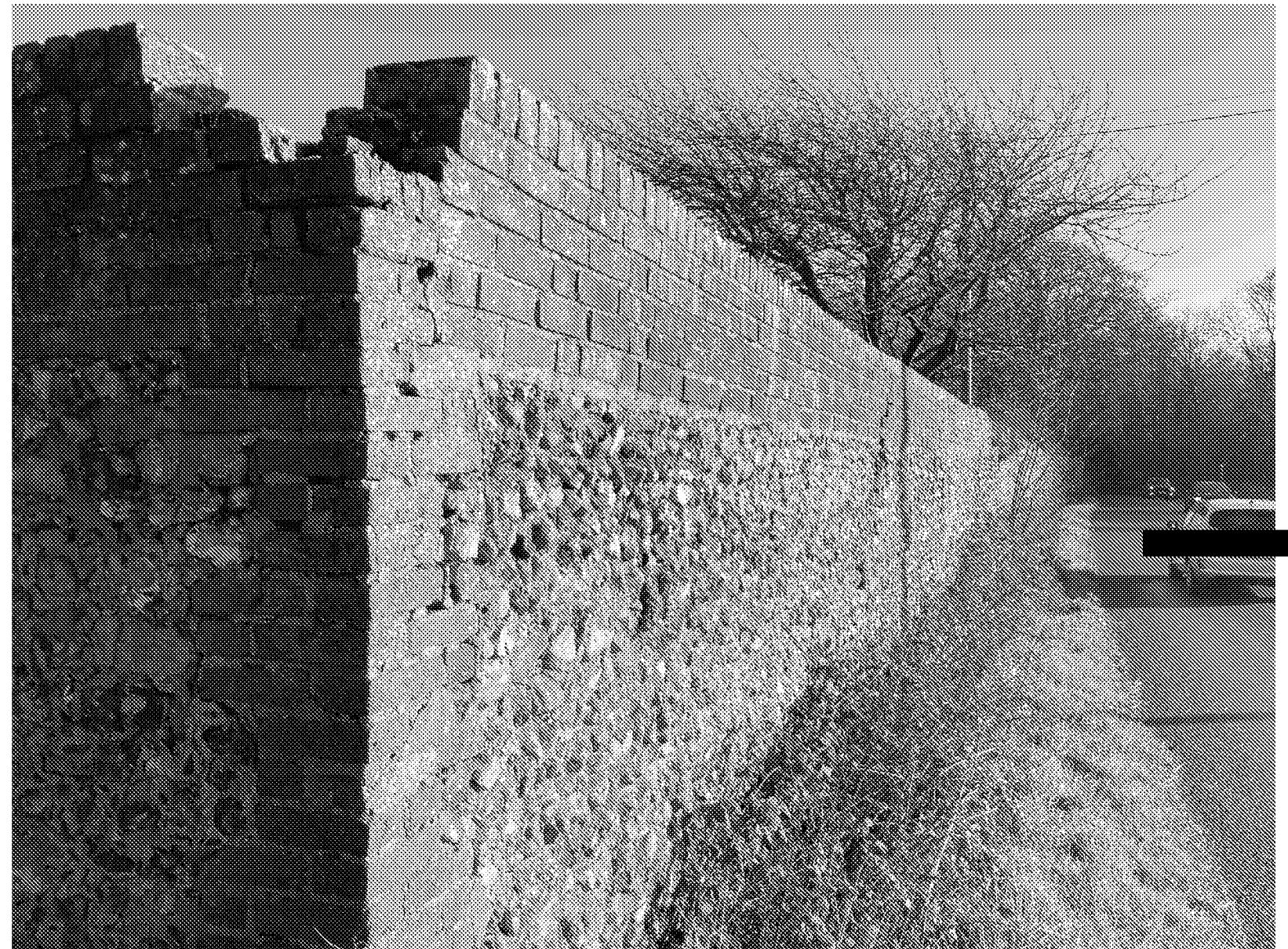
03 Existing Nyton House Boundary Wall
