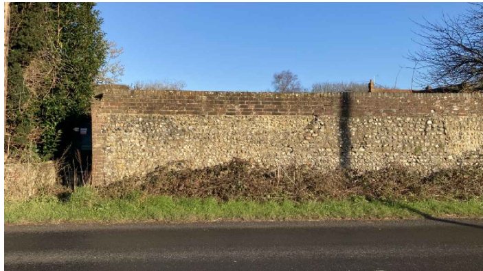
Photo 5 - The extent of the wall as seen from Nyton Road, looking north
