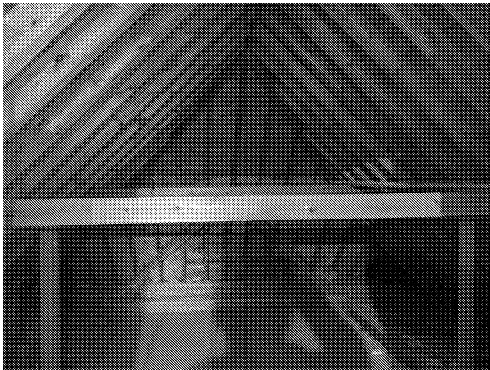
Photograph No. 05 - Other loft areas of Building B1 are still open to the rafters.
