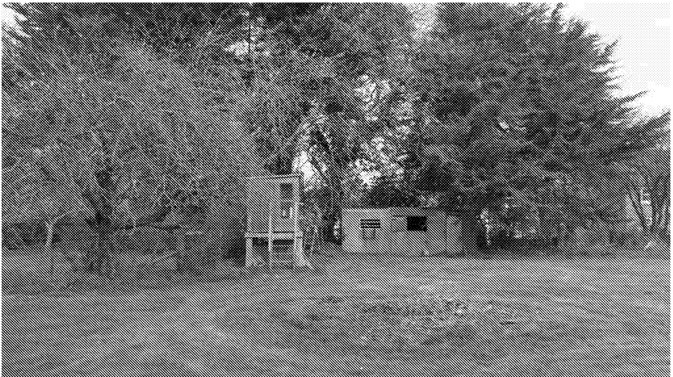
Photograph No. 10 - Buildings B02 and B03 offering 'negligible' bat roost potential.
