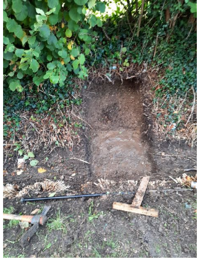
Hole for the headwall
