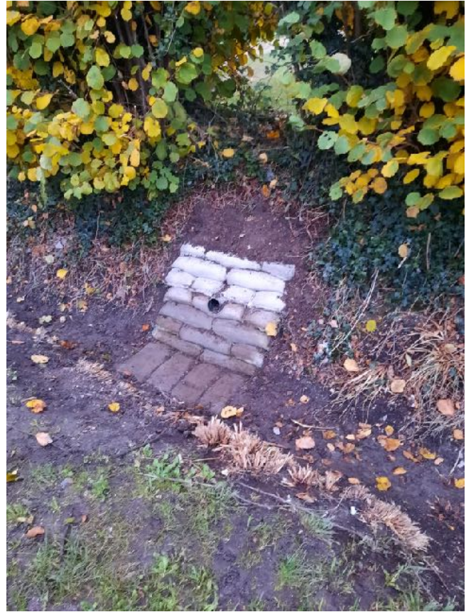
View of the headwall and ditch and completed headwall backfilled
