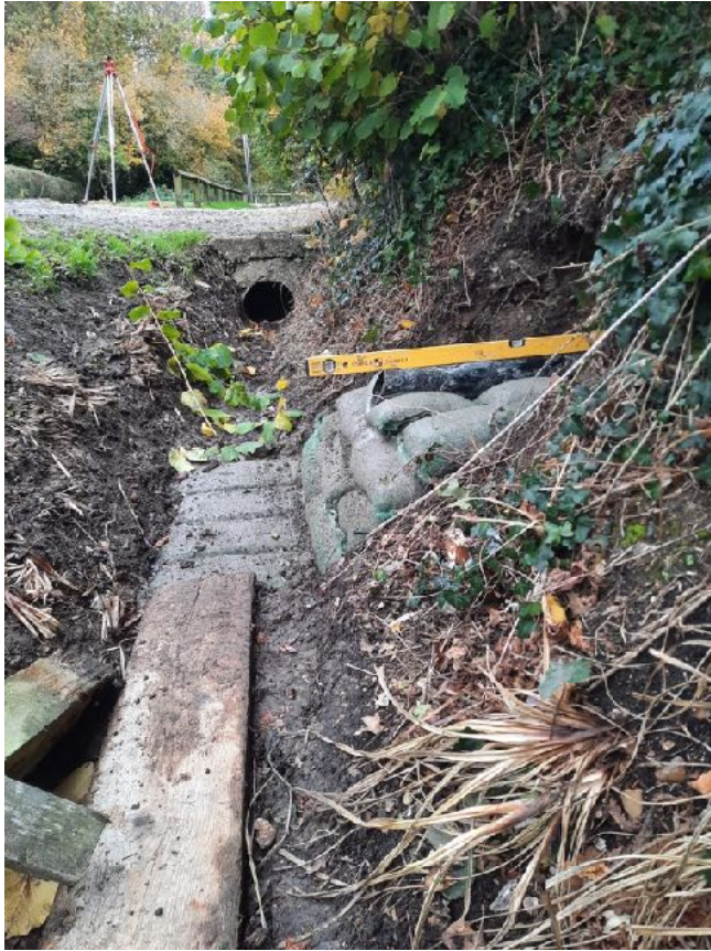
View of the headwall and ditch and completed headwall backfilled
