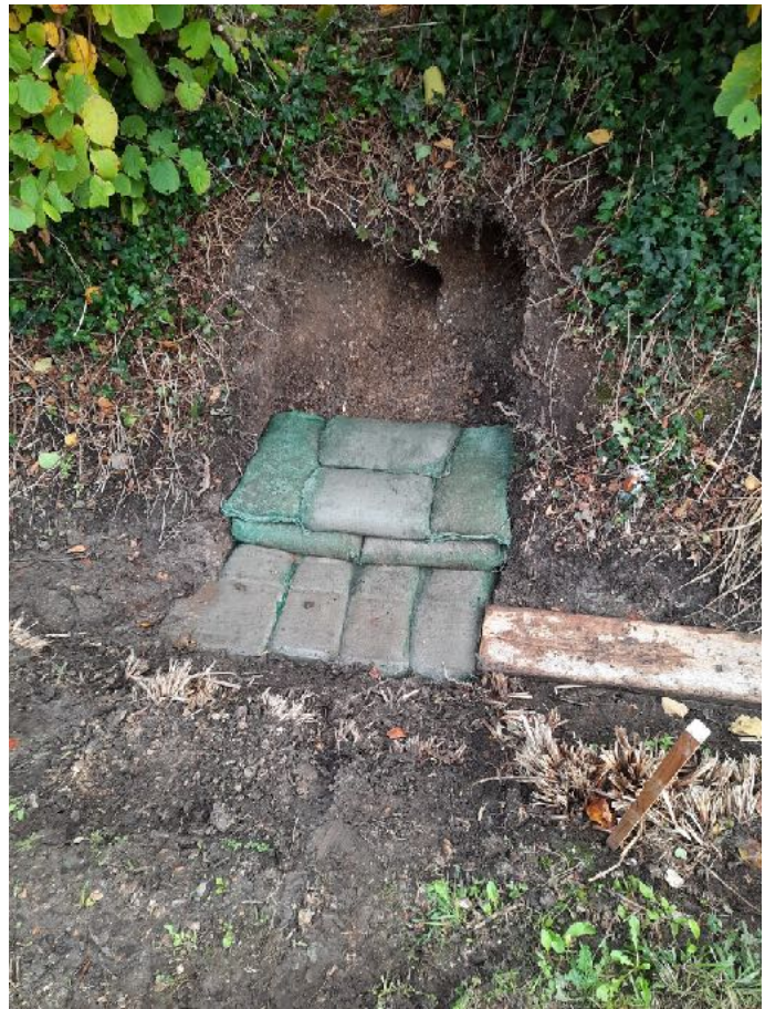
Base sandbags in place, secured with reinforcement bars
