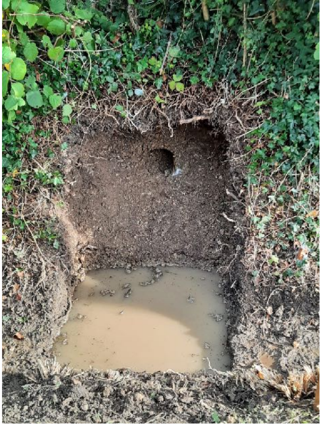
Hole for the headwall
