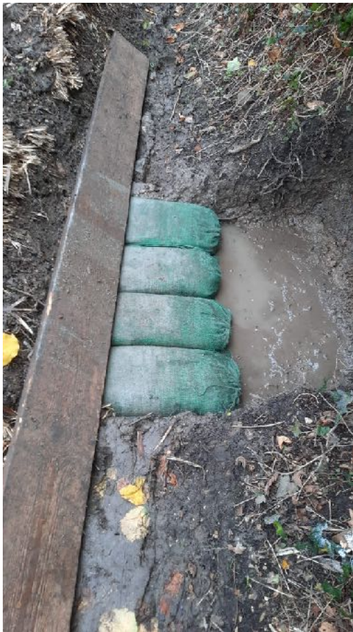
Base sandbags in place, secured with reinforcement bars
