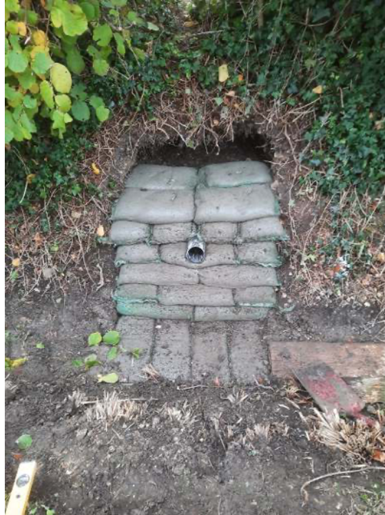
Completed Bagwork Headwall with 150mm dia. Outlet Pipe
