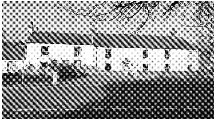
Figure 12: Argyl House (left) and The Long House (right) along Nyton Road
