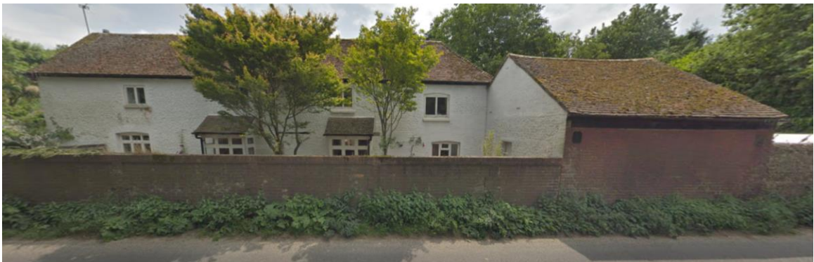
Figure 1.2 – Nyton Lodge (Source: Google Earth)
