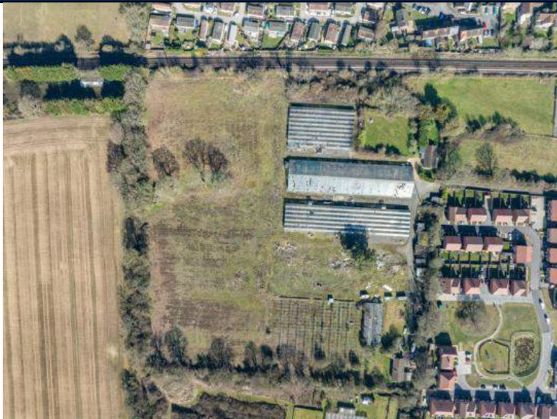
Aerial image of the site prior to the removal of the outbuildings
