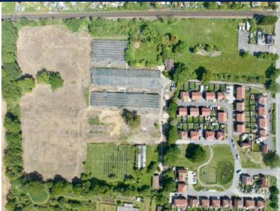
Aerial image of the site following removal of the outbuildings
