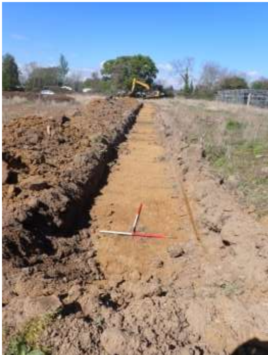
Plate 32: Trench F, from the south
