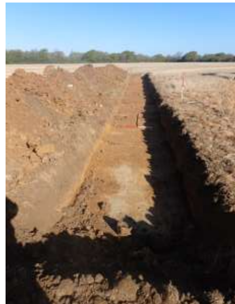
Plate 4: Trench 2, from the north-west
