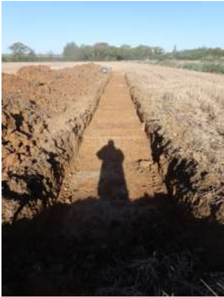
Plate 1: Trench 1, from the east
