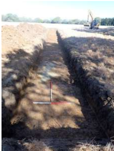
Plate 8: Trench 5, from the south-east
