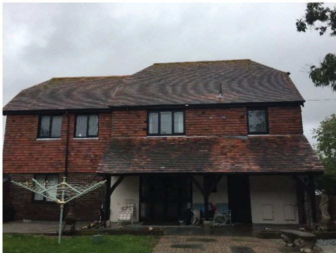
Photograph 4 Western elevation of Building 1
