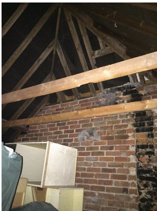
Photograph 1 Building 1 roof void
