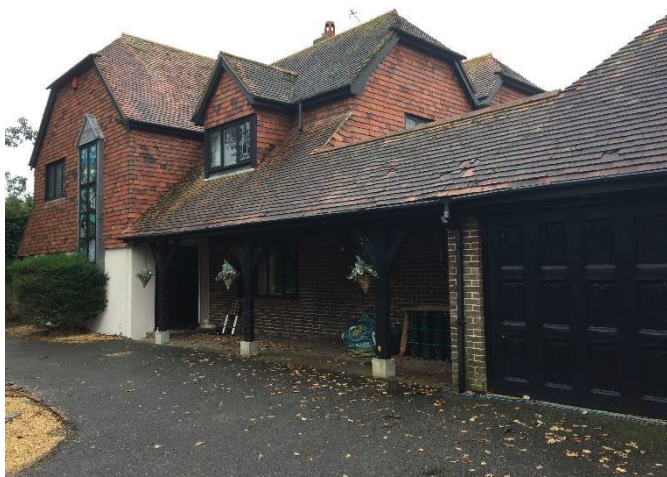
Photograph 2 Eastern and northern elevations of Building 1
