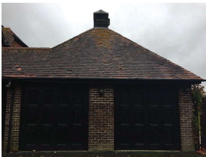
Photograph 3 Eastern elevation of Building 2
