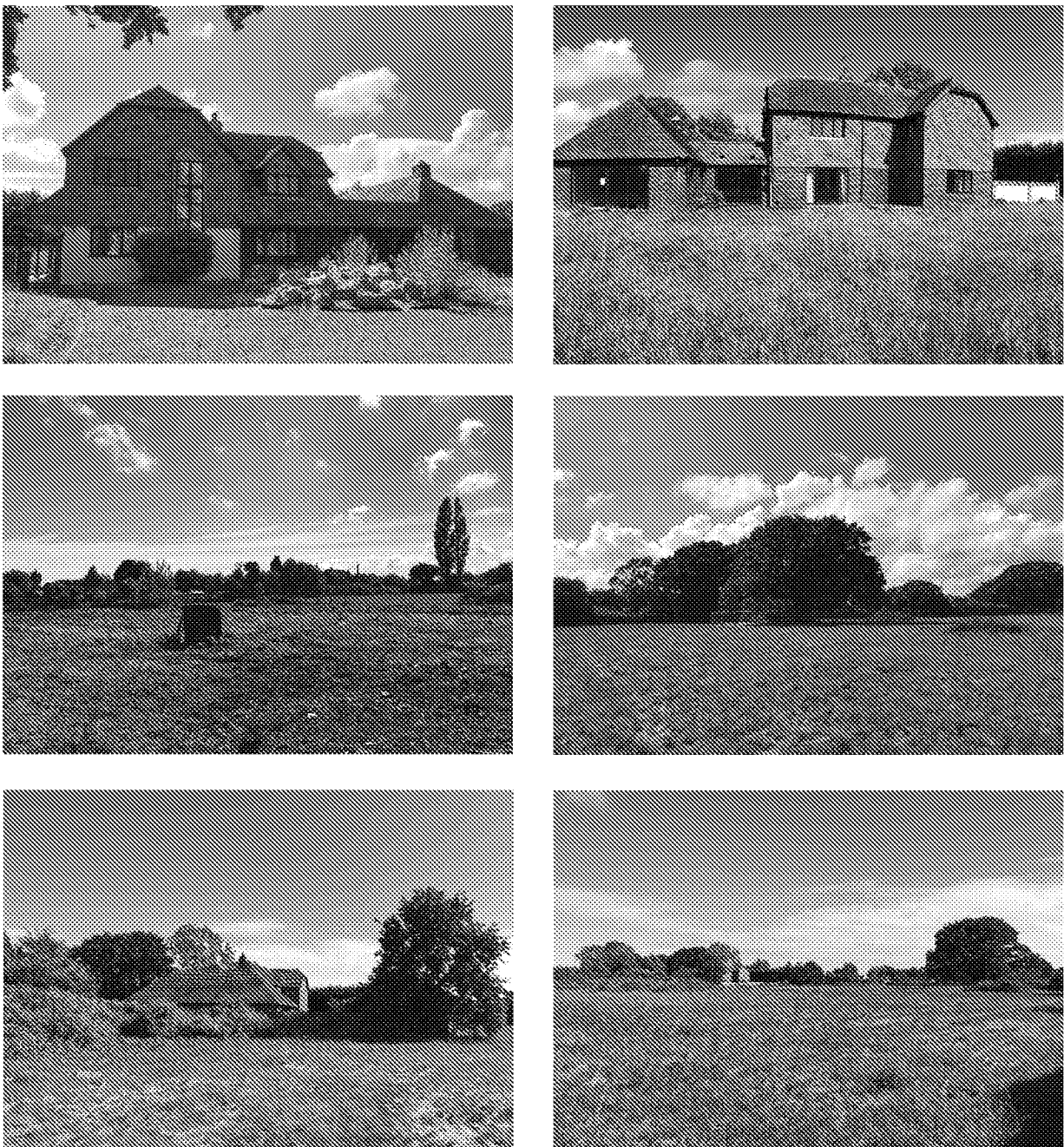
Images of the site and existing building
