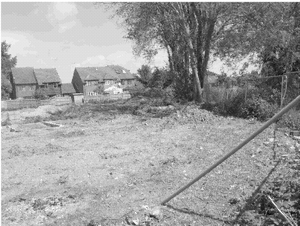
Building site to the east of Swan Court flats where four houses will be erected
