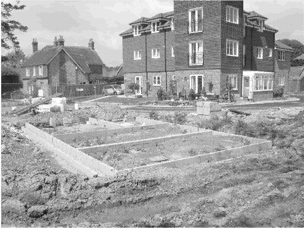
Plot 4 partly constructed
