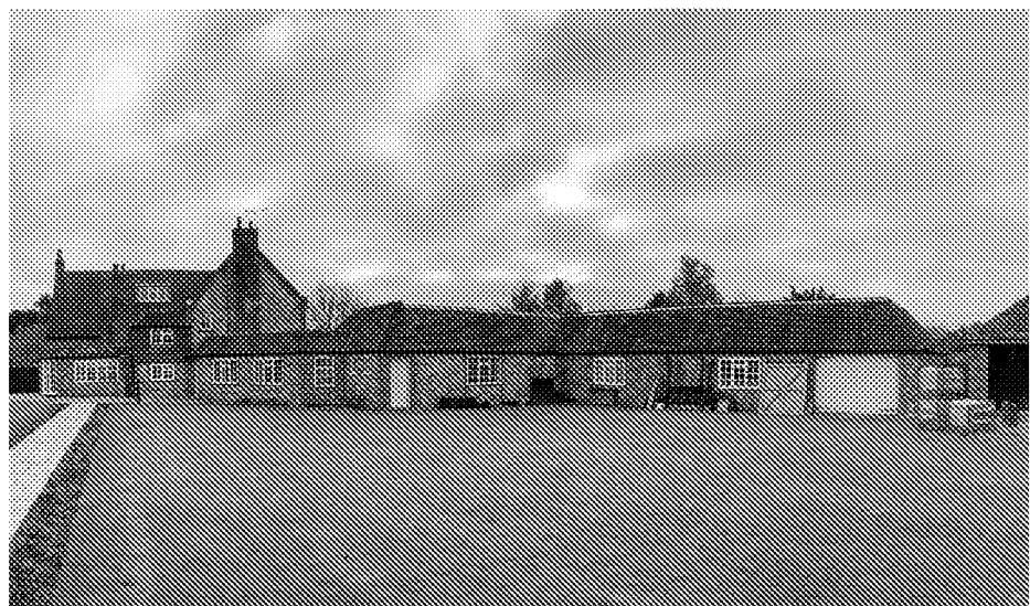
view of north and west elevation
