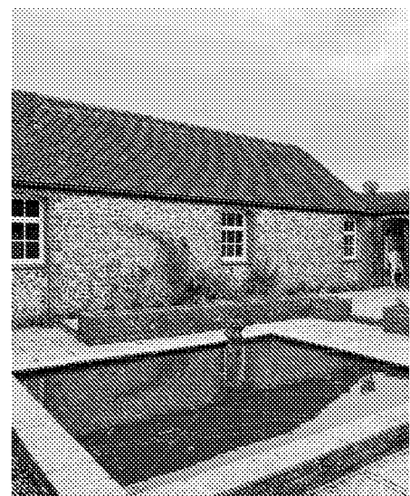
view of east elevation
