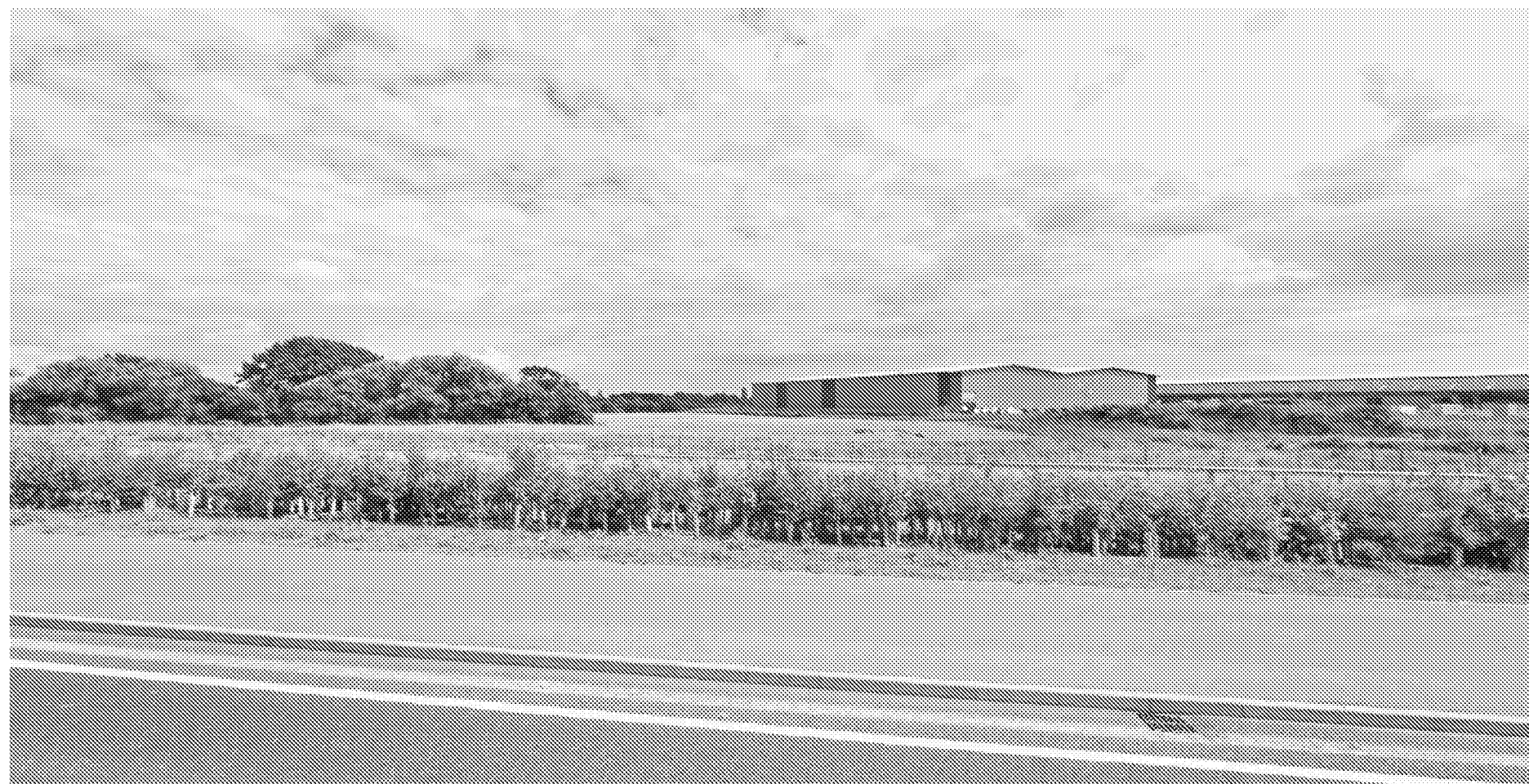
View onto the existing Rolls Royce development and the site with its existing trees towards its left as seen from the BNRR
