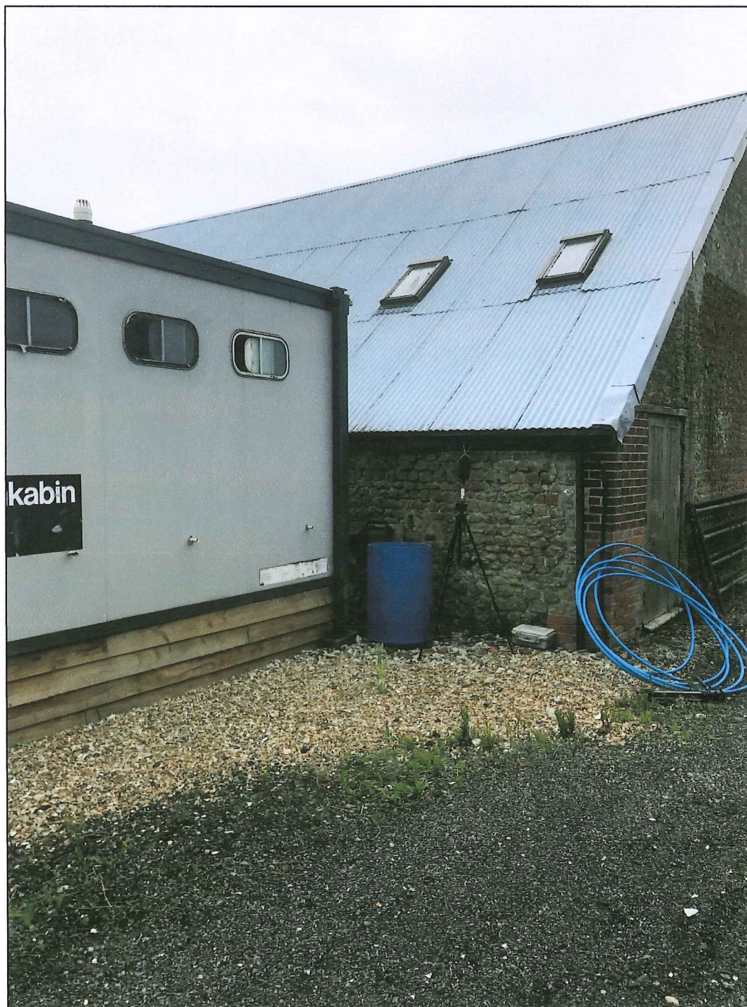
Looking west at rear of Lidsey Barn
