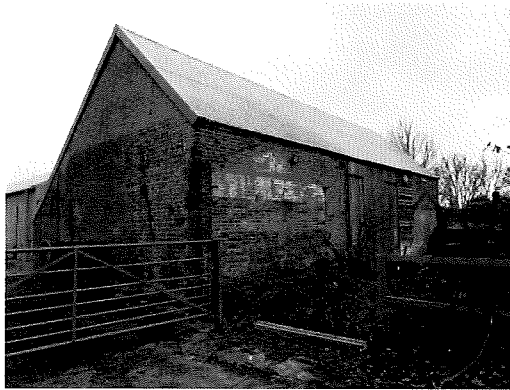
West facing frontage and northern end
