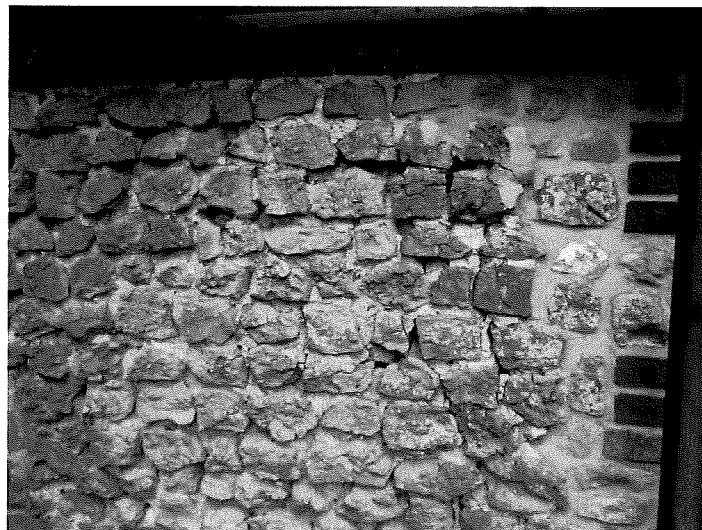
Low rear wall facing west showing crevices where mortar had been lost
