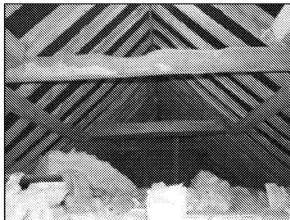
The roof, looking west.
