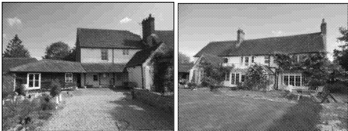
The south elevation of the house, viewed from the south-west (above left) and from the south-east (above right),
