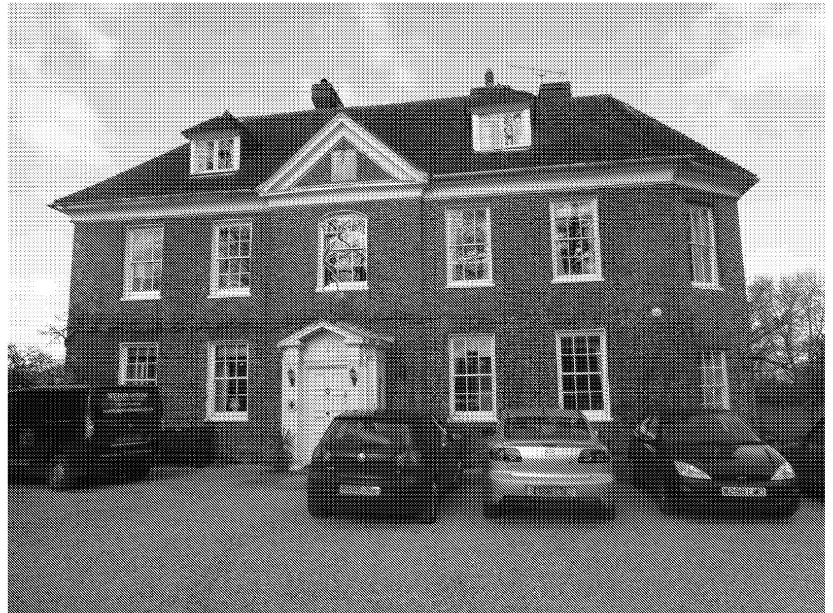
03: Main entrance of Nyton House (South Elevation)
