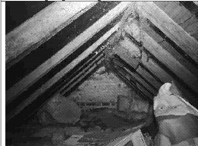
Photo 9: Cottage roof void
