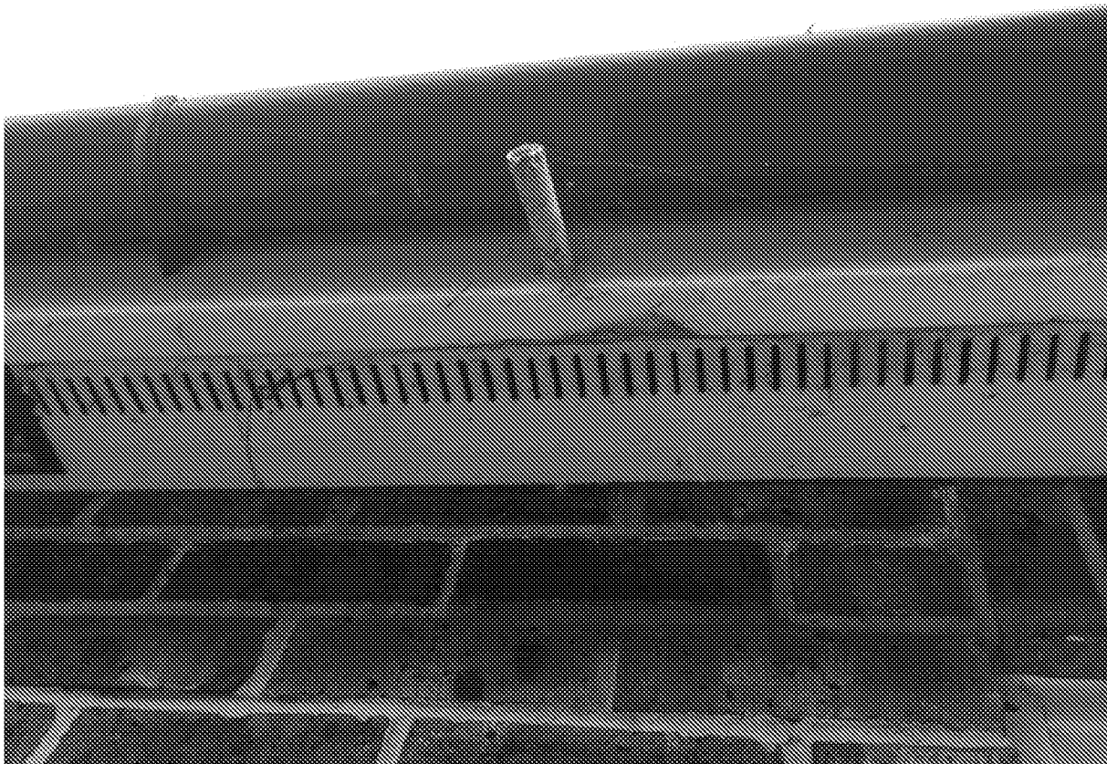
Figure 17. The vented plastic soffits are tight fitting with no suitable roosting crevices present.
