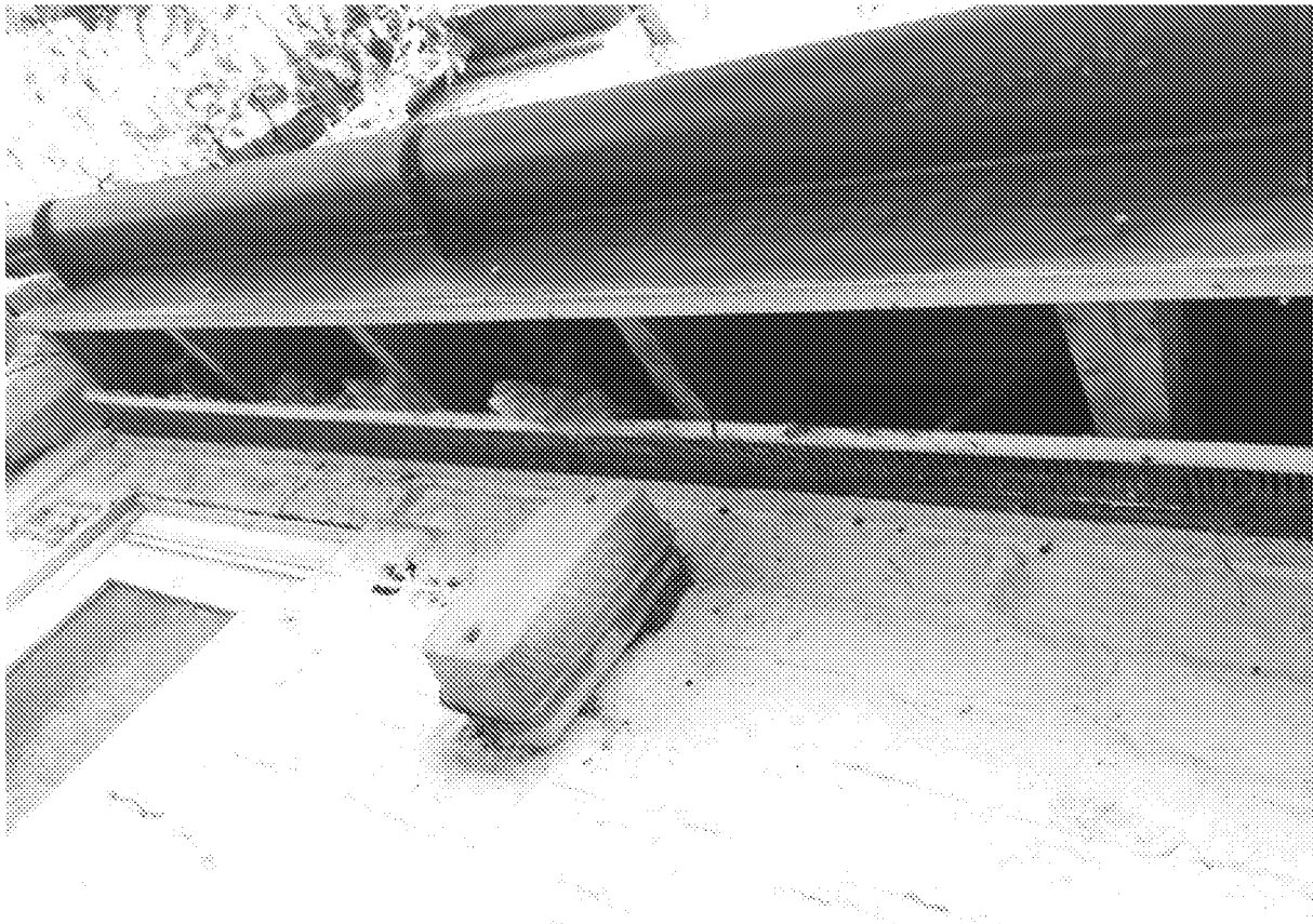
Figure 22. The wooden soffit box, on the single-story extension on the southern face, which is missing the bottom board leading to direct access to a cavity with bitumen lining which is stiffed with rockwool insulation.
