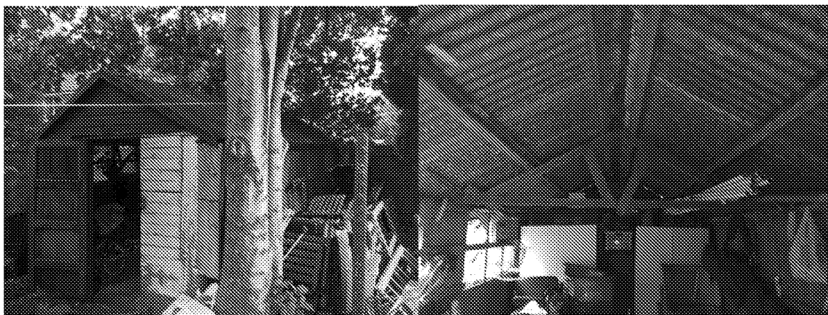
Figure 19. The wooden shiplap shed with a corrugated metal roof.
