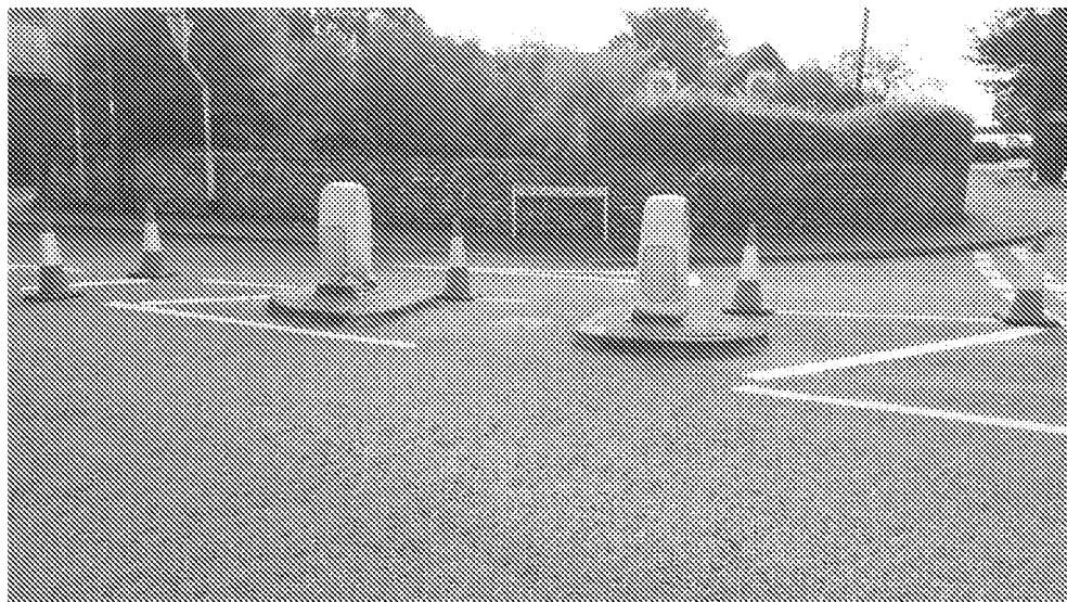
Photograph 3 Pedestrian crossing, Fontwell Avenue
