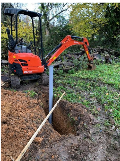
Winter Ground Water Dates and Image of installation of monitoring pipe (1 of 2 pipes installed) (See drawing 17-1179-PL 401A for location)
