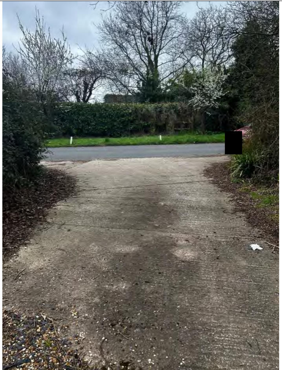
Photograph 23: Hardstanding access to the south- west of site
