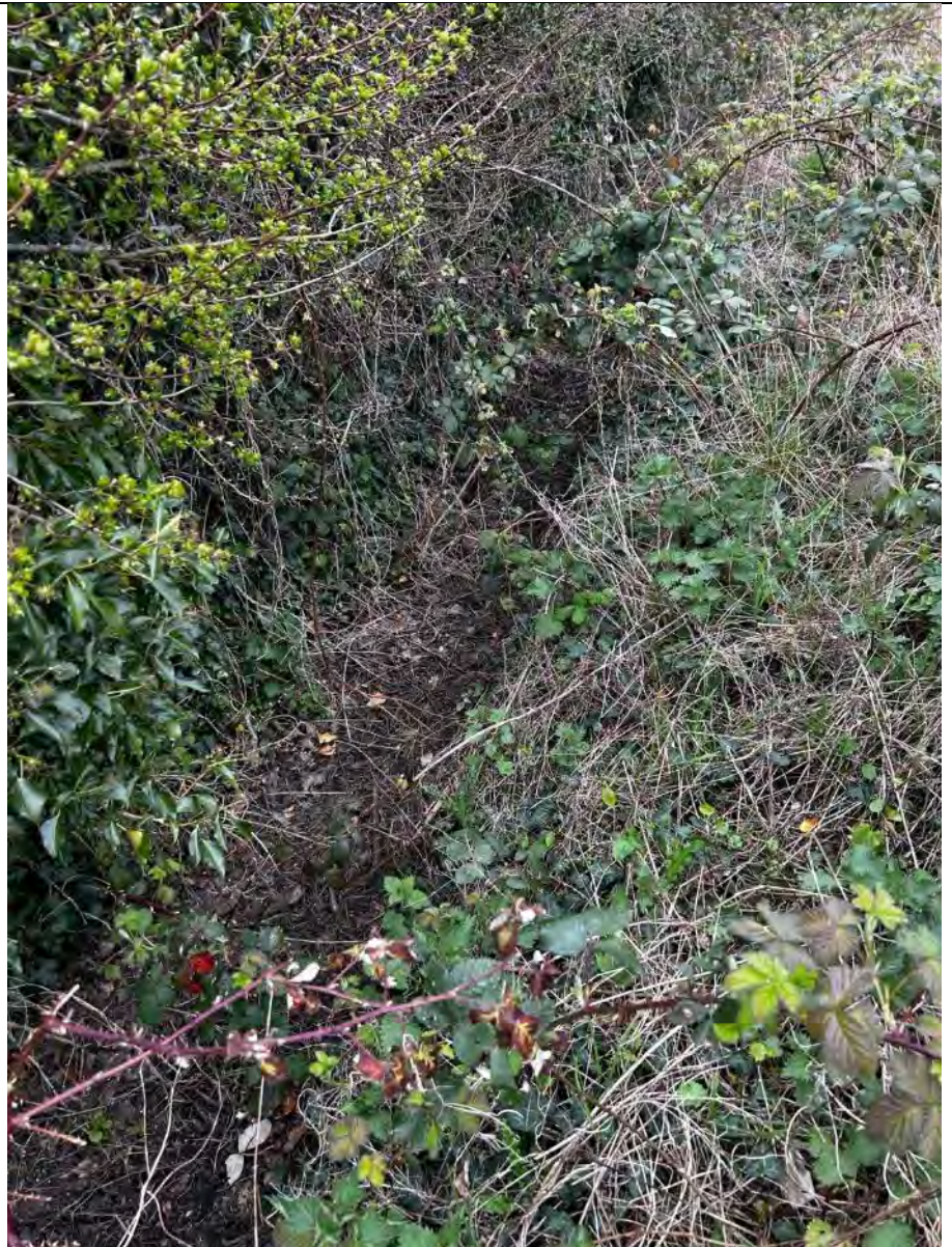
Photograph 17: Dry ditch running along the north of site
