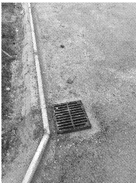
Road gully constructed within visitor parking bays opposite Plot 7 (during construction, prior to surface course application)
