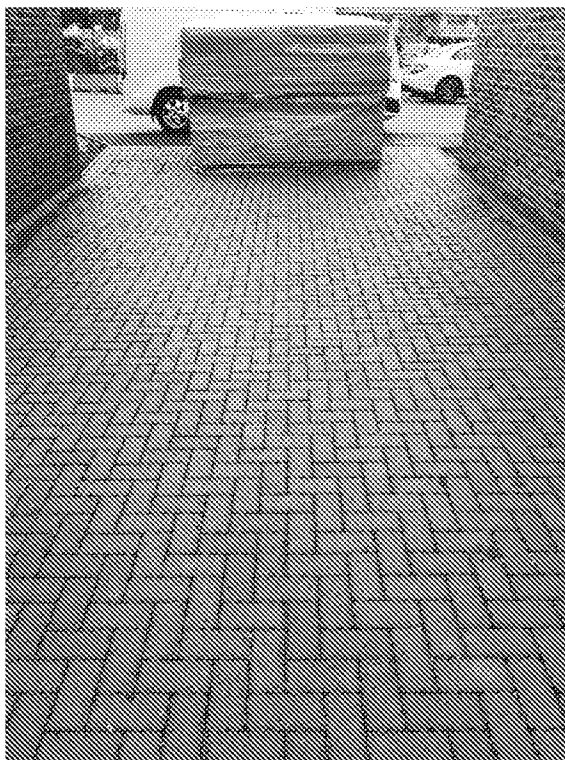
Permeable Paving at Plot 16 and Plot 17 shared driveway
