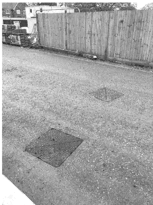
Manholes F16 (left) and S17 (right)
