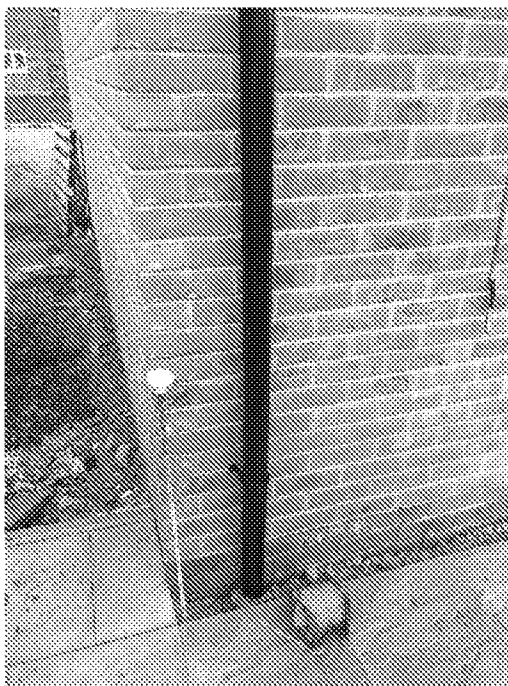
Rainwater pipe at Plot 8
