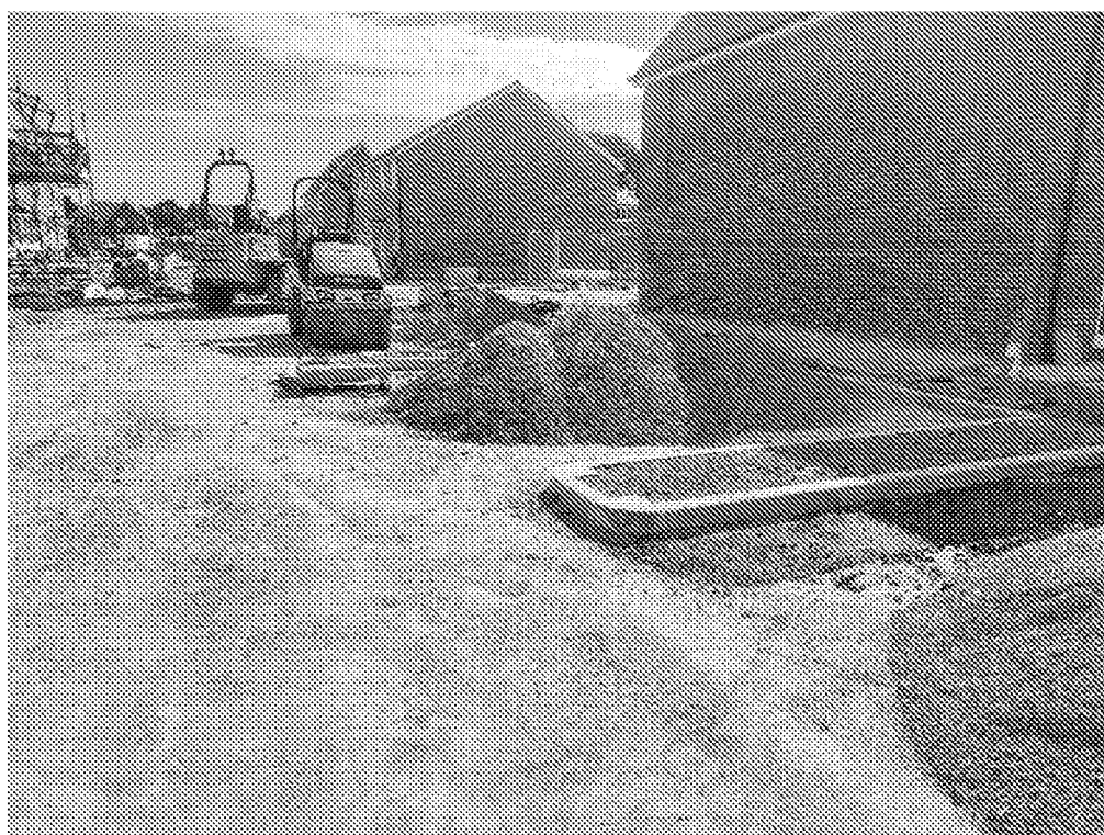
Preparation of permeable paved area adjacent to Plots 51 and 52 (during construction)
