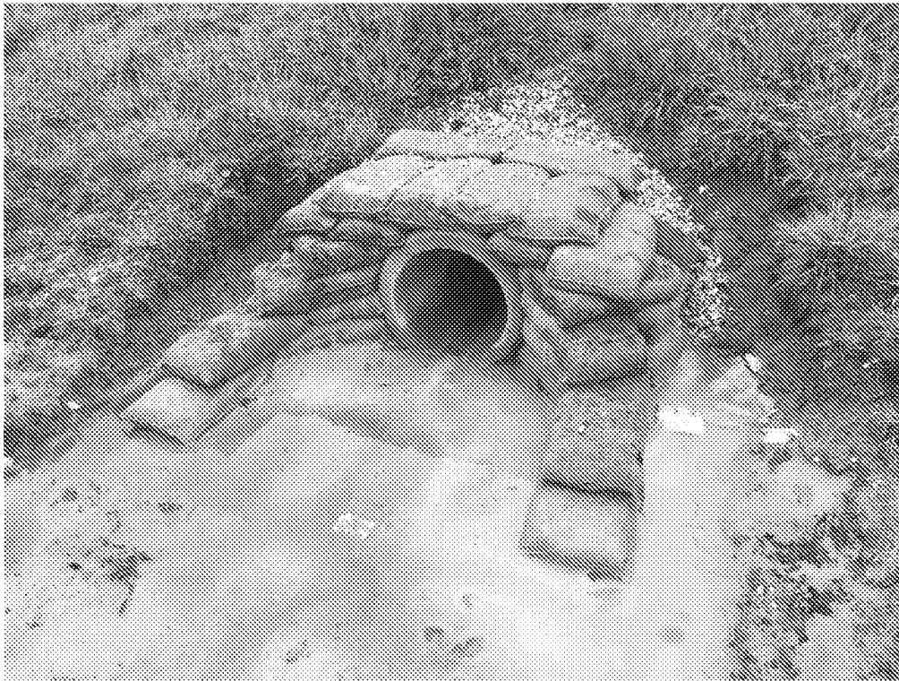
Inlet/Outlet Pipe and Headwall
