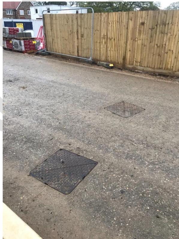
Manholes F16 (left) and S17 (right)
