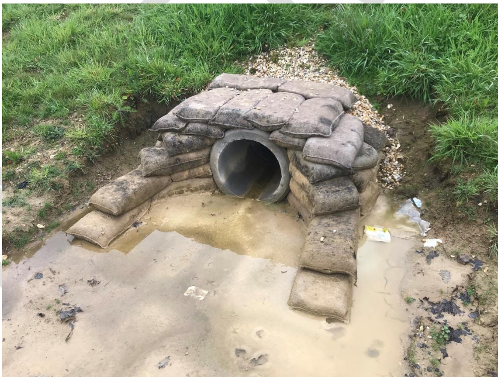
Inlet/Outlet Pipe and Headwall
