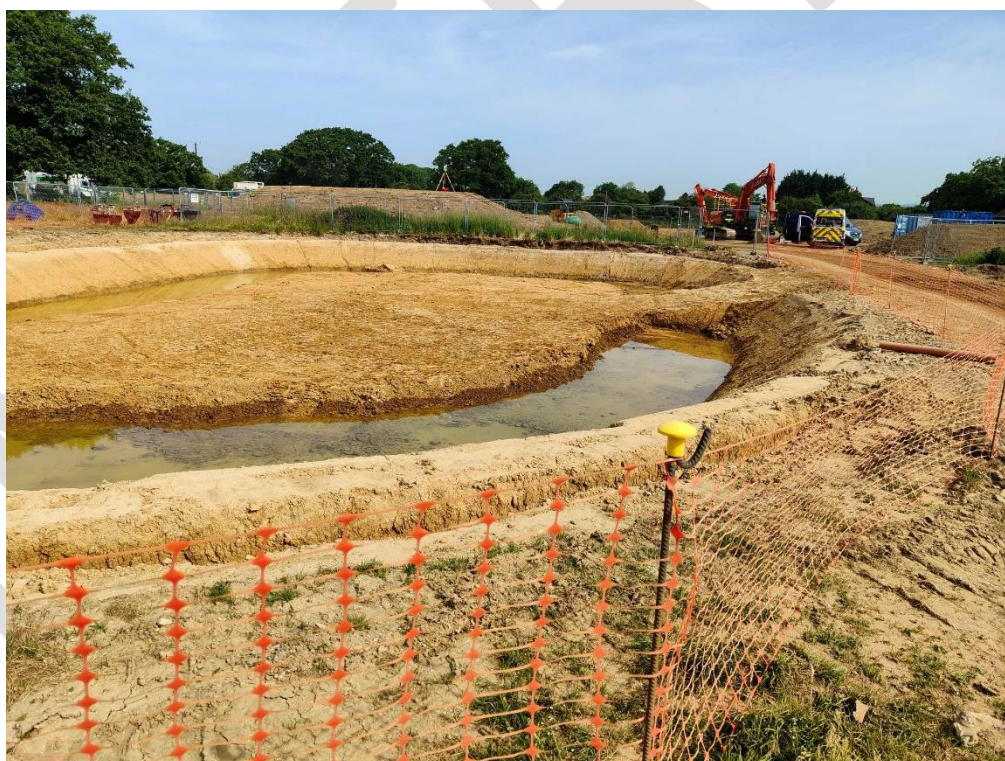
Attenuation Basin during formation, and confirmation of high groundwater (during construction)
