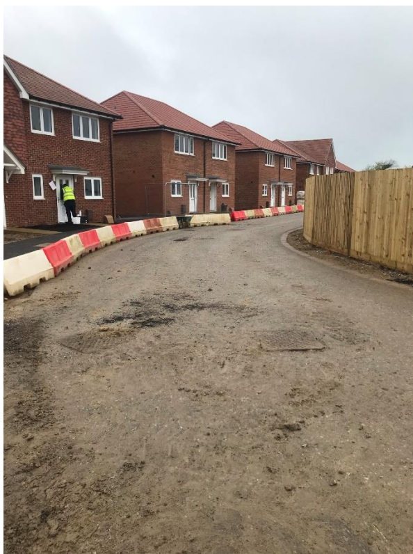
Manholes F17 (left) and S18 (right)
