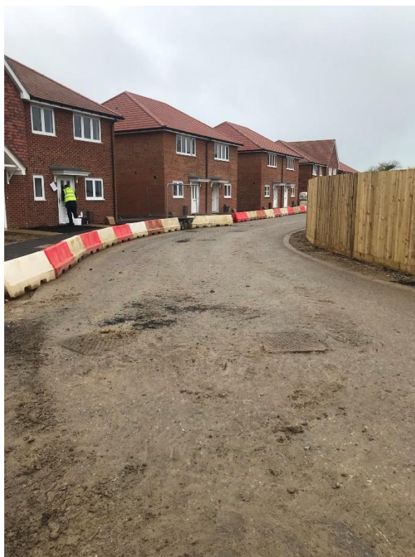
Manholes F17 (left) and S18 (right)
