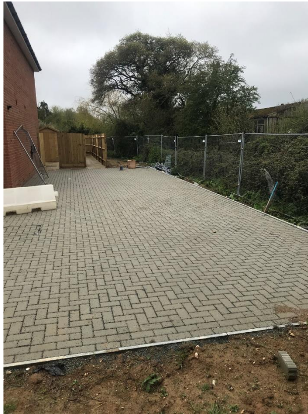
Permeable Paving at Plot 20 and Plot 21 shared driveway
