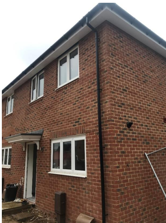
Rainwater pipe at Plot 18 (roof level – during construction)
