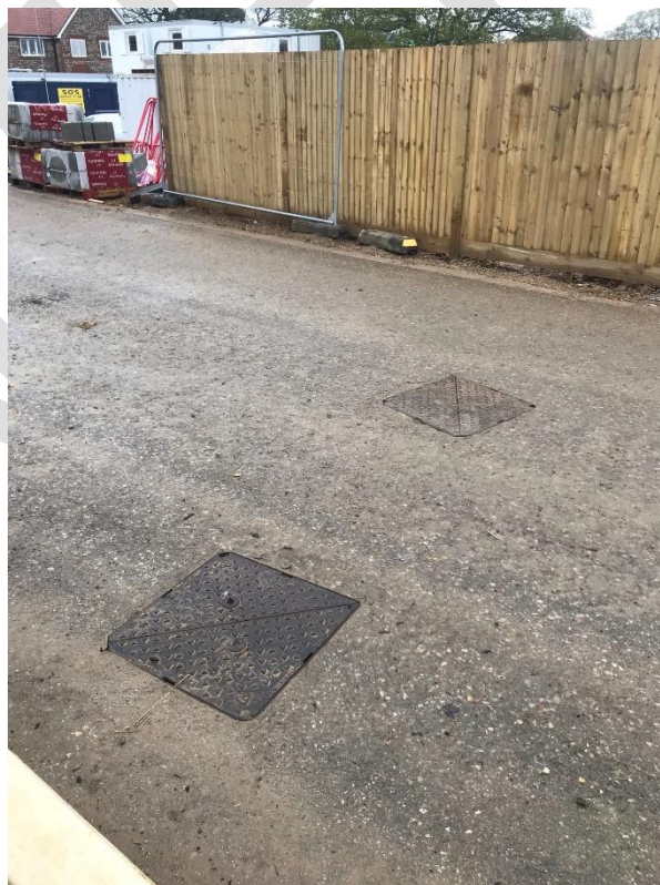
Manholes F16 (left) and S17 (right)
