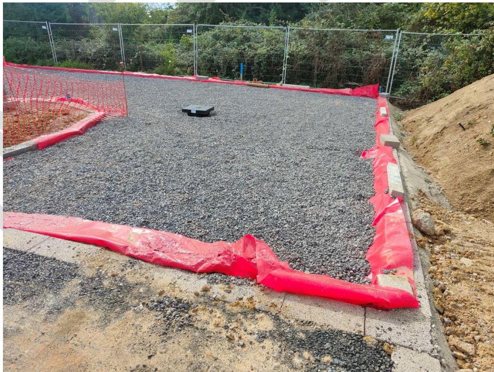
Confirmation of permeable paving membrane/liner and sub-base material at Plot 20 and Plot 21 shared driveway (during construction)
