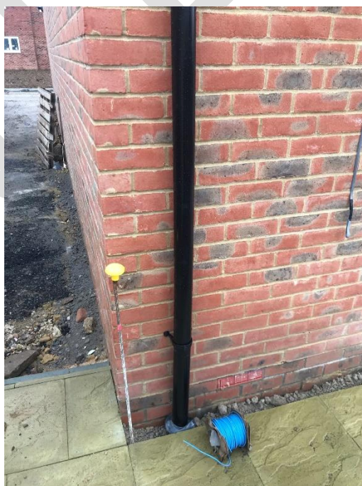
Rainwater pipe at Plot 8
