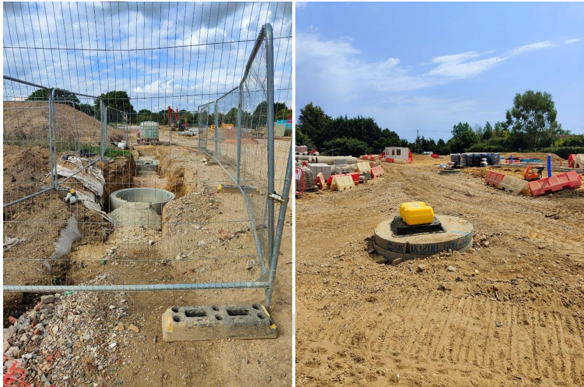
Example manholes on site (during construction)
