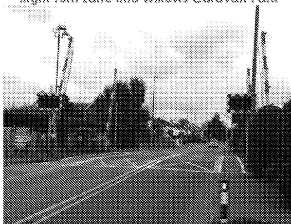
Woodgate Level crossing
