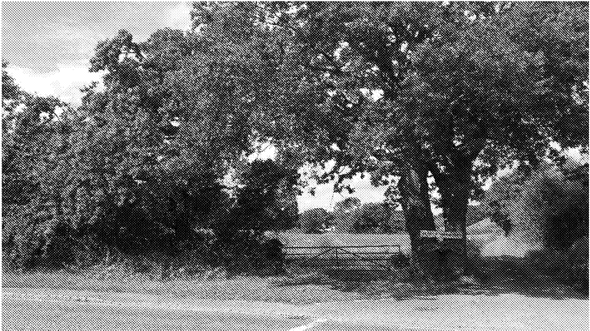
Existing northern access into site (with field gate) – proposed to be the secondary access point.
