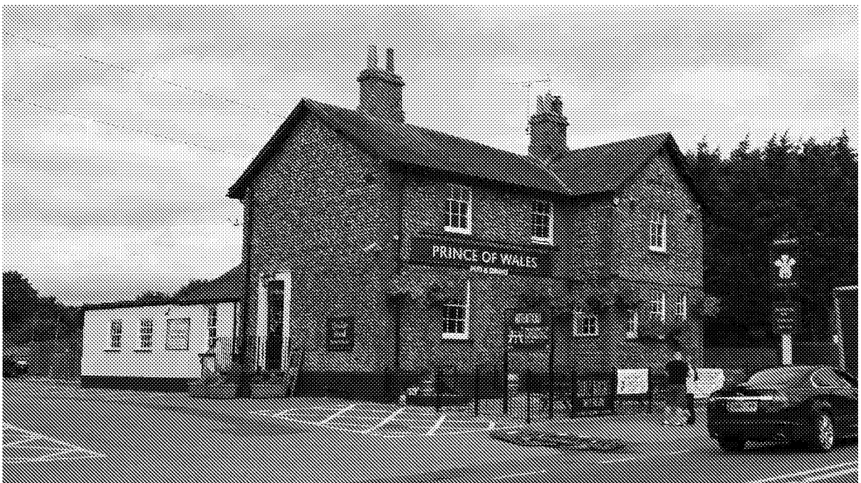
Prince of Wales put, adjacent to the northeast corner of the site.
