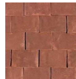
ROOF CLAY TILES
