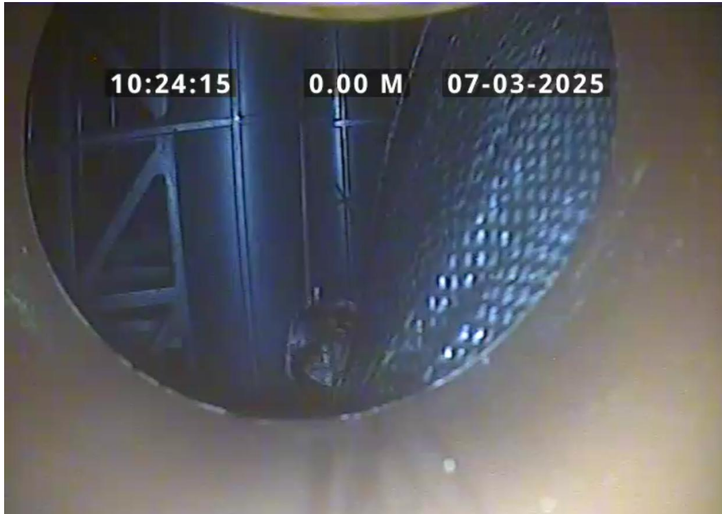
Start node, manhole, reference: PSCP165
