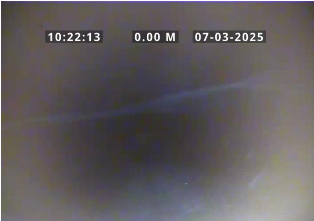
Start node, manhole, reference: PSCP160
