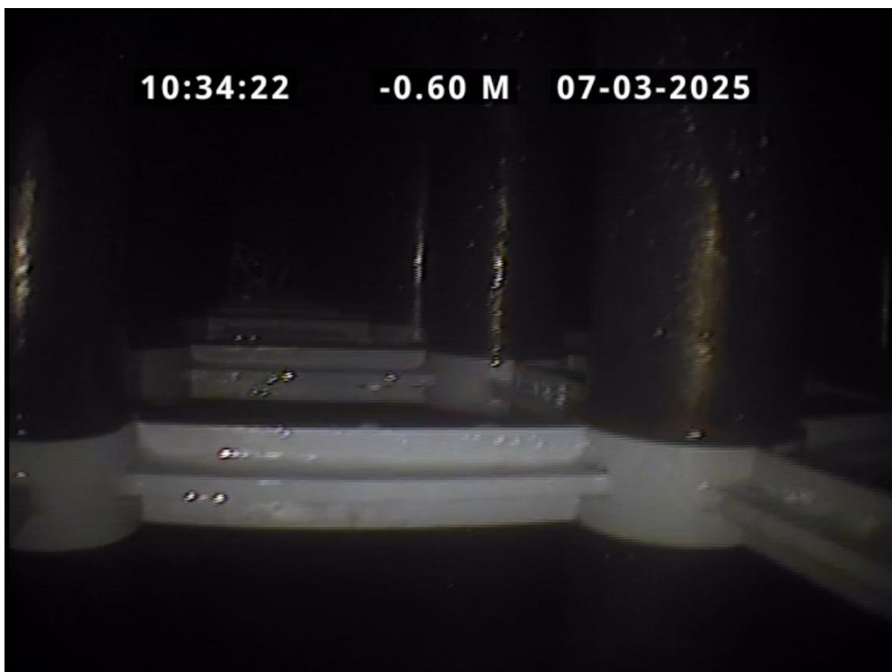
Finish node, soakaway, reference: SA6-7
