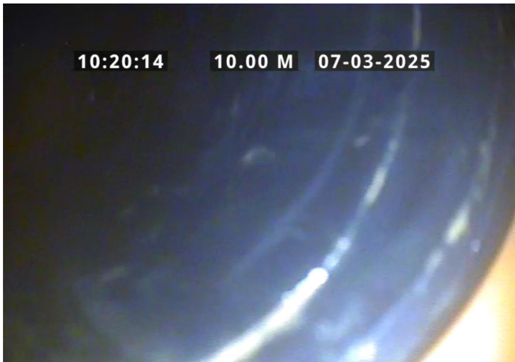
Finish node, manhole, reference: PSCP160
