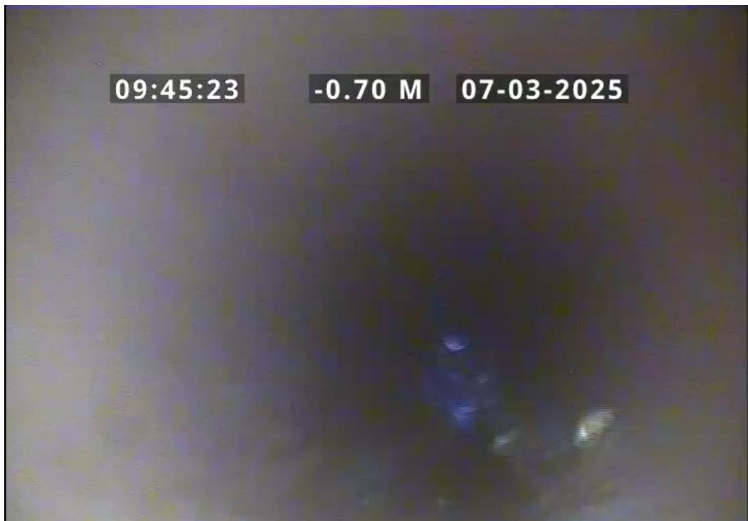
Start node, manhole, reference: PS23
