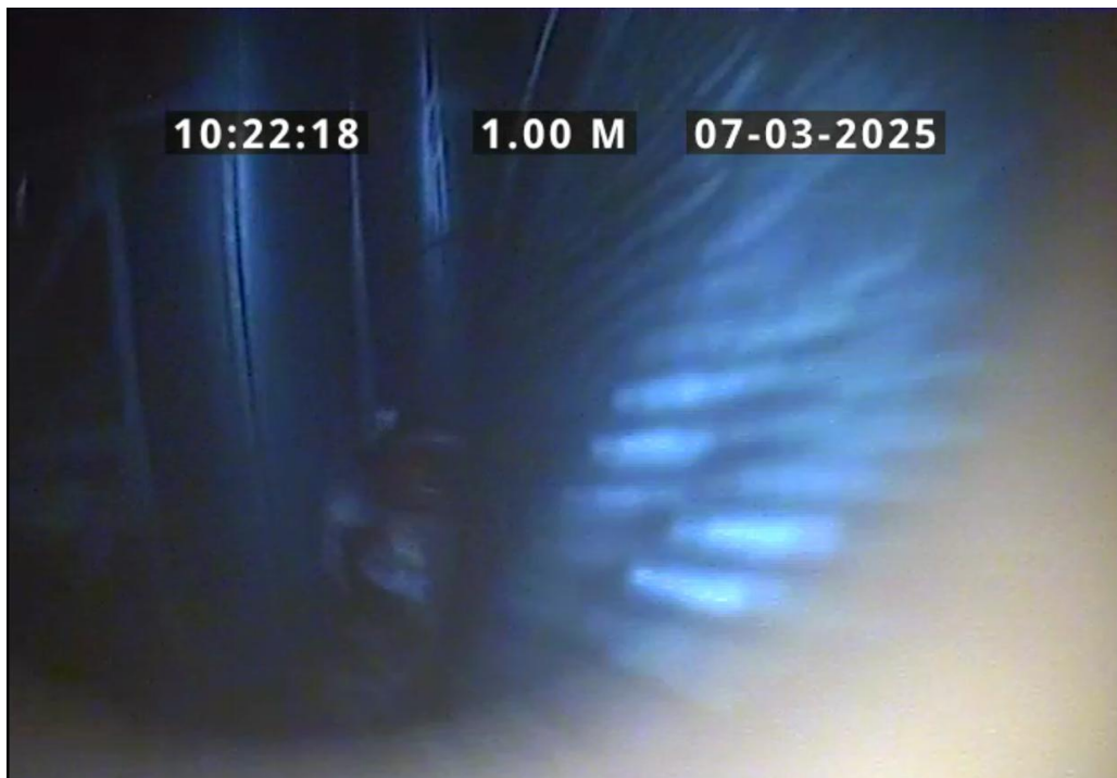
Finish node, soakaway, reference: SA9-11
