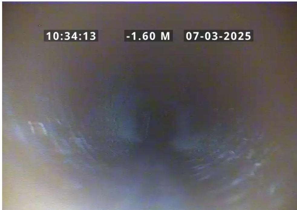
Start node, manhole, reference: PSCP170
