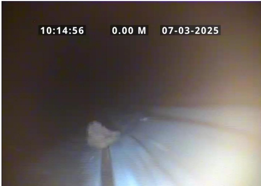
Start node, manhole, reference: PS5279
