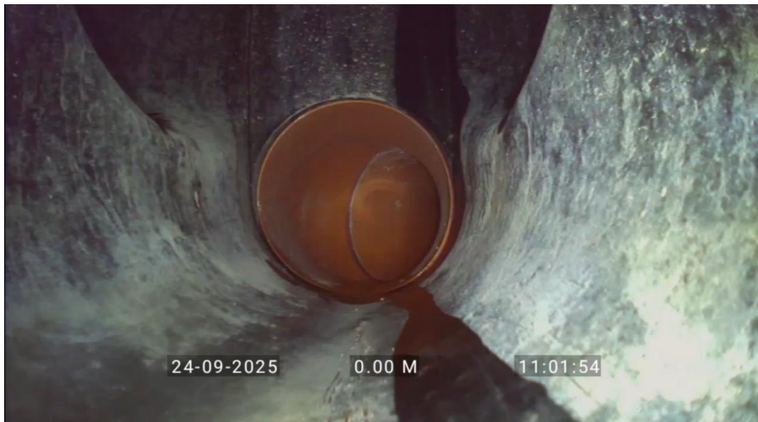
Start node, manhole, reference: PS291
