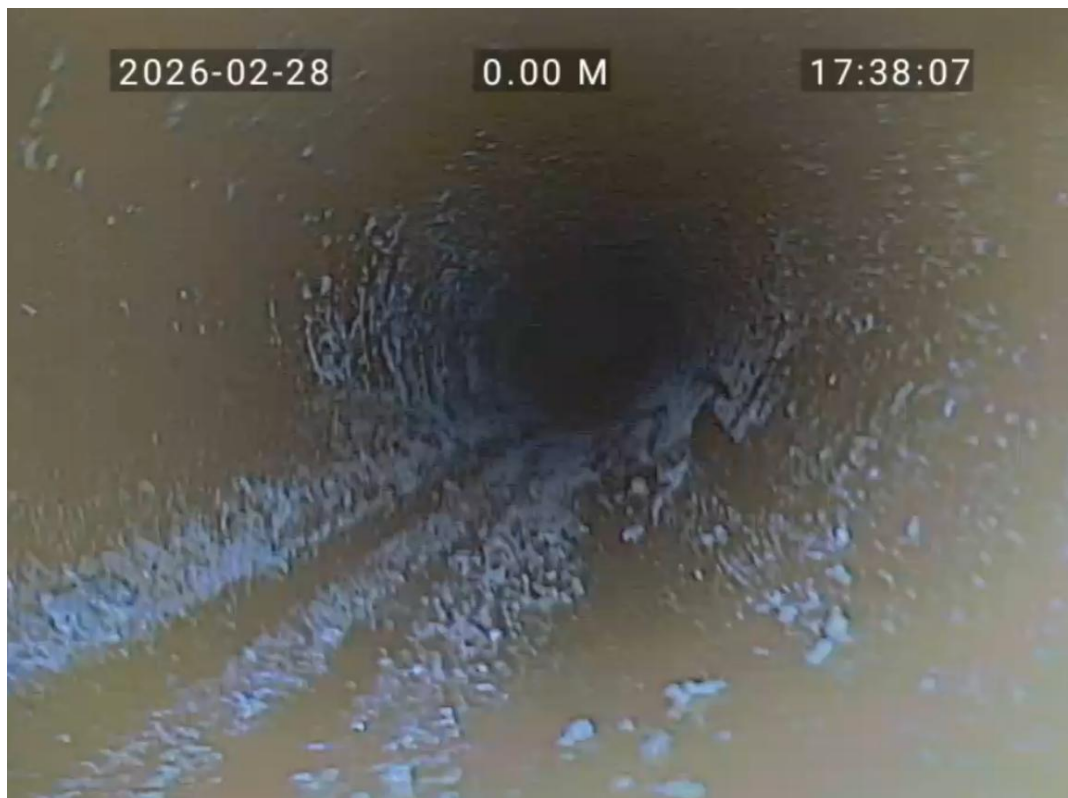
Start node, manhole, reference: PS275
