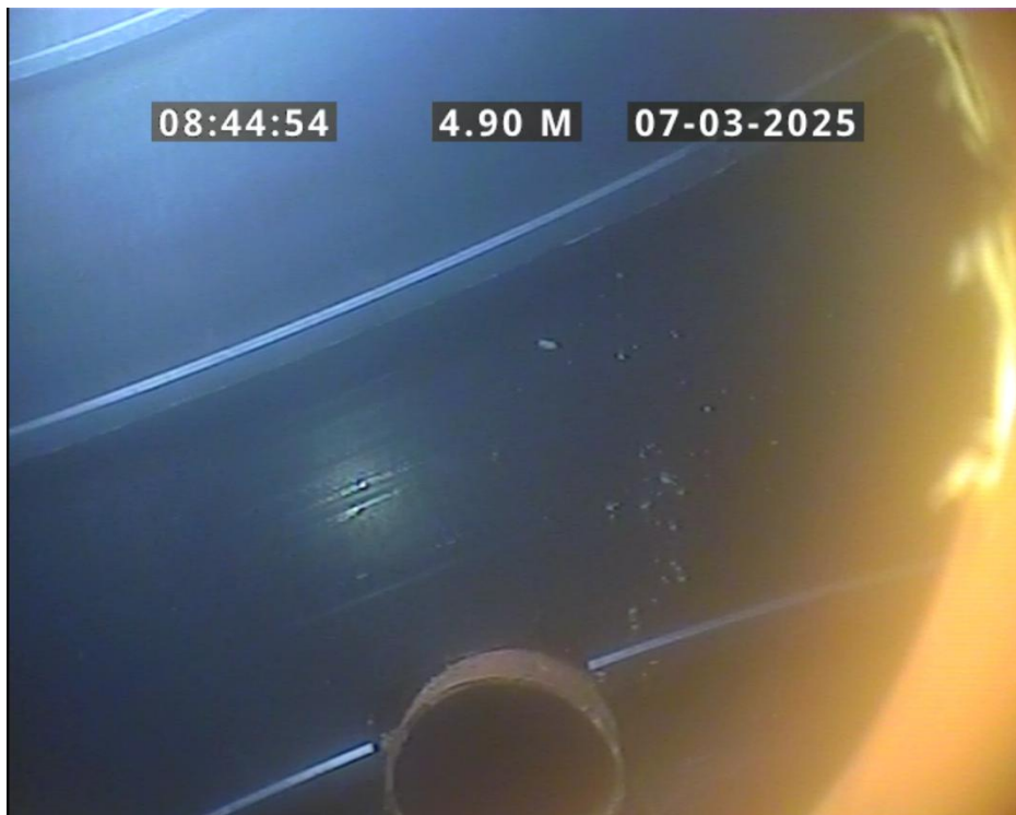
Finish node, manhole, reference: PSCP67
