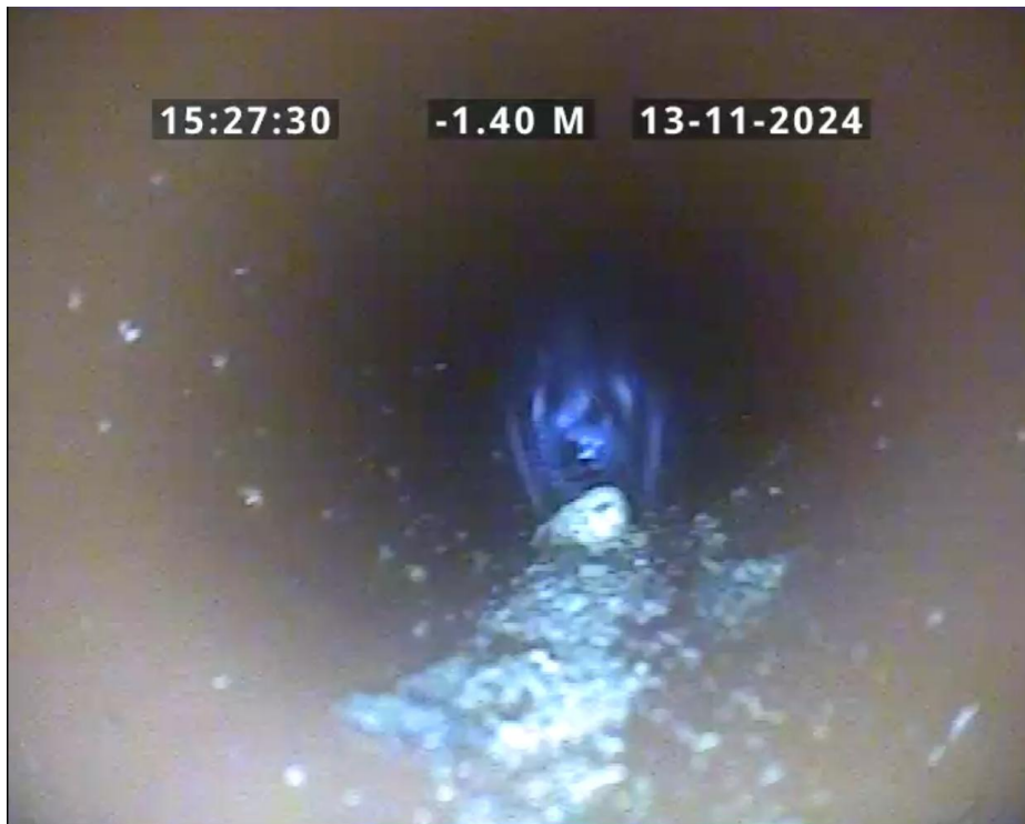
Start node, manhole, reference: PSCP5301
