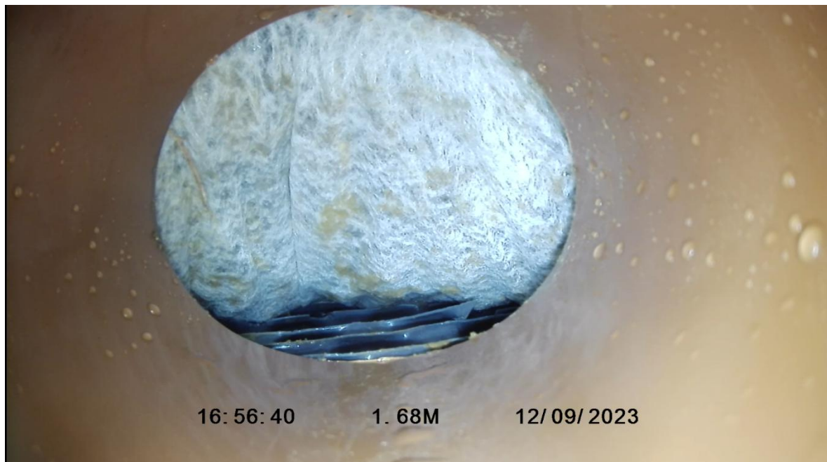
Finish node, soakaway, reference: SA52
