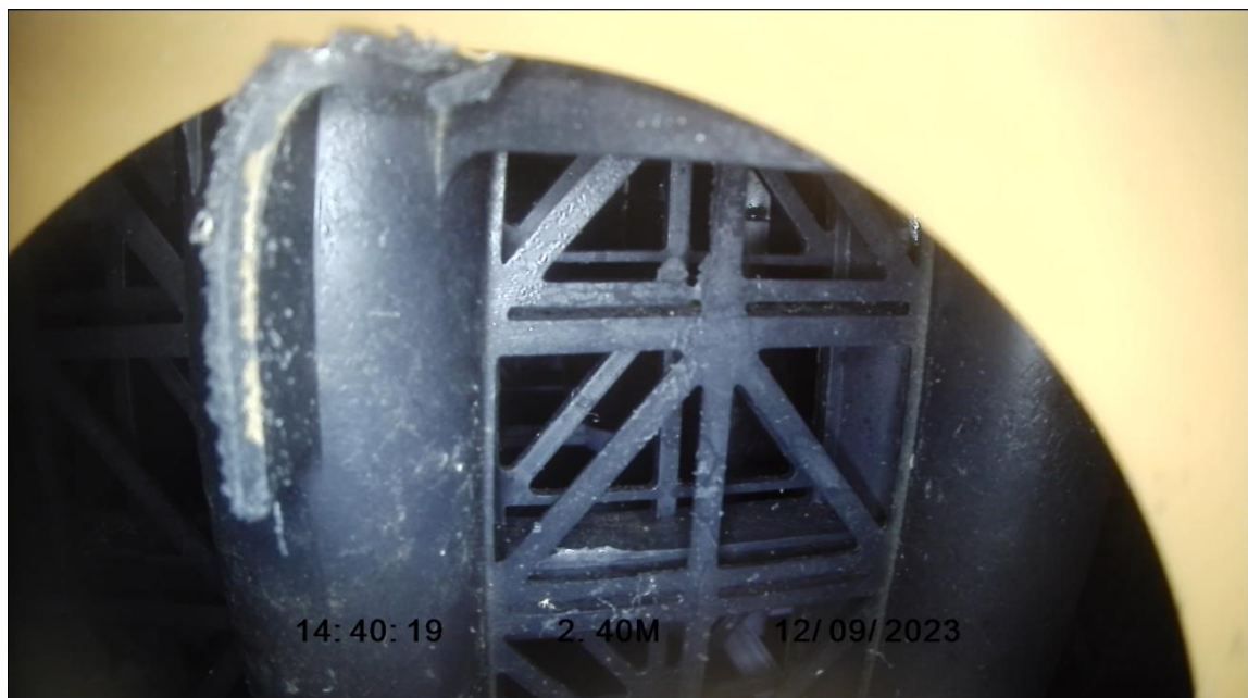
Finish node, soakaway, reference: SA43-45
