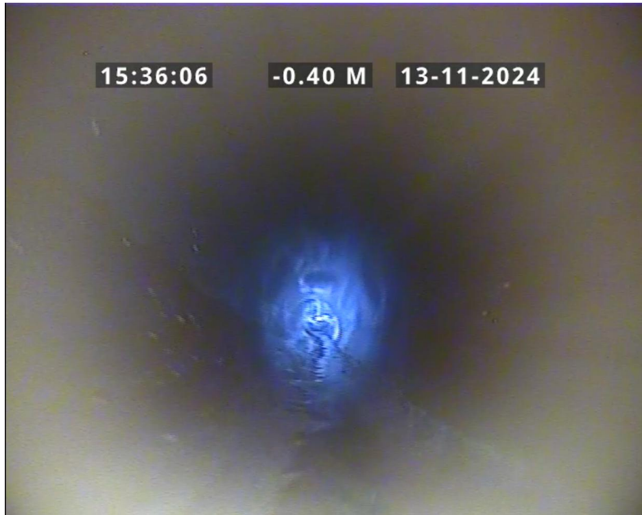
Start node, manhole, reference: PS5283
