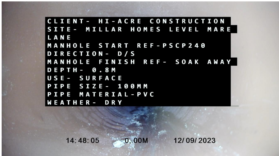
Start node, manhole, reference: PSCP240
