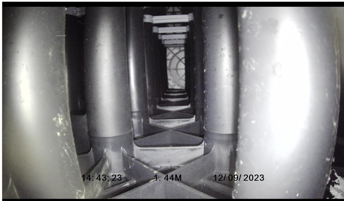
Finish node, soakaway, reference: SA40-42
