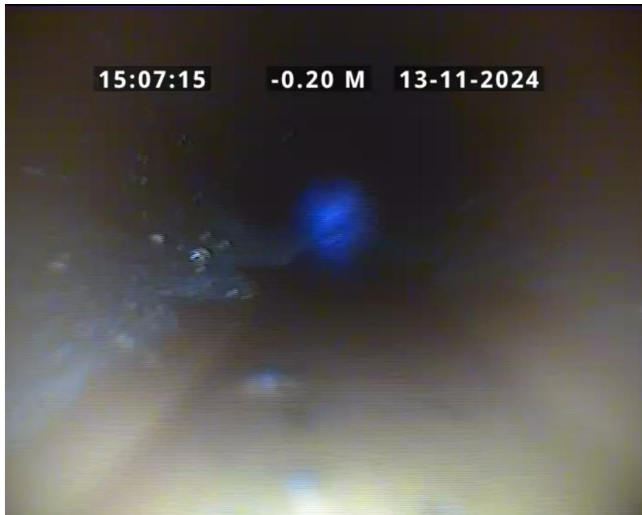
Start node, manhole, reference: PS243
