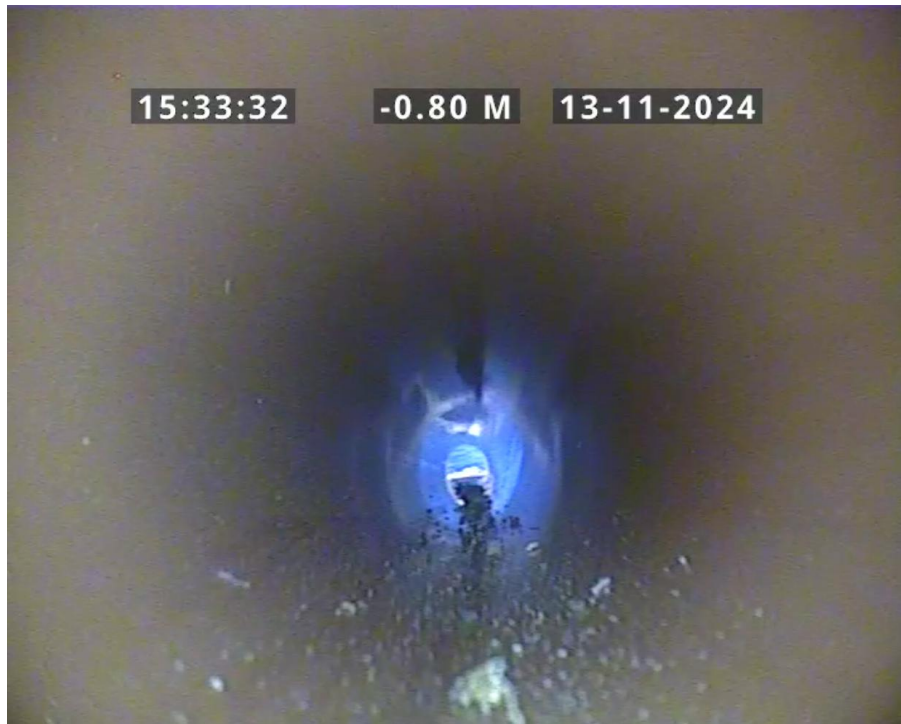
Start node, manhole, reference: PS298
