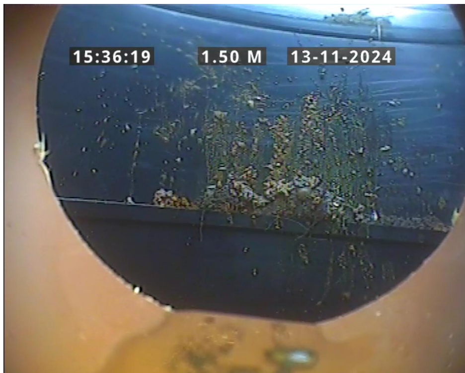
Finish node, manhole, reference: PSCP231
