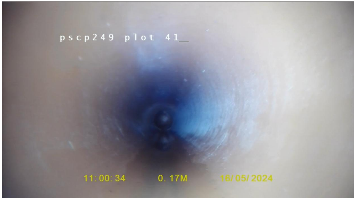
Start node, manhole, reference : PSCP249
