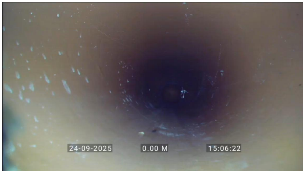
Start node, manhole, reference: PS54
