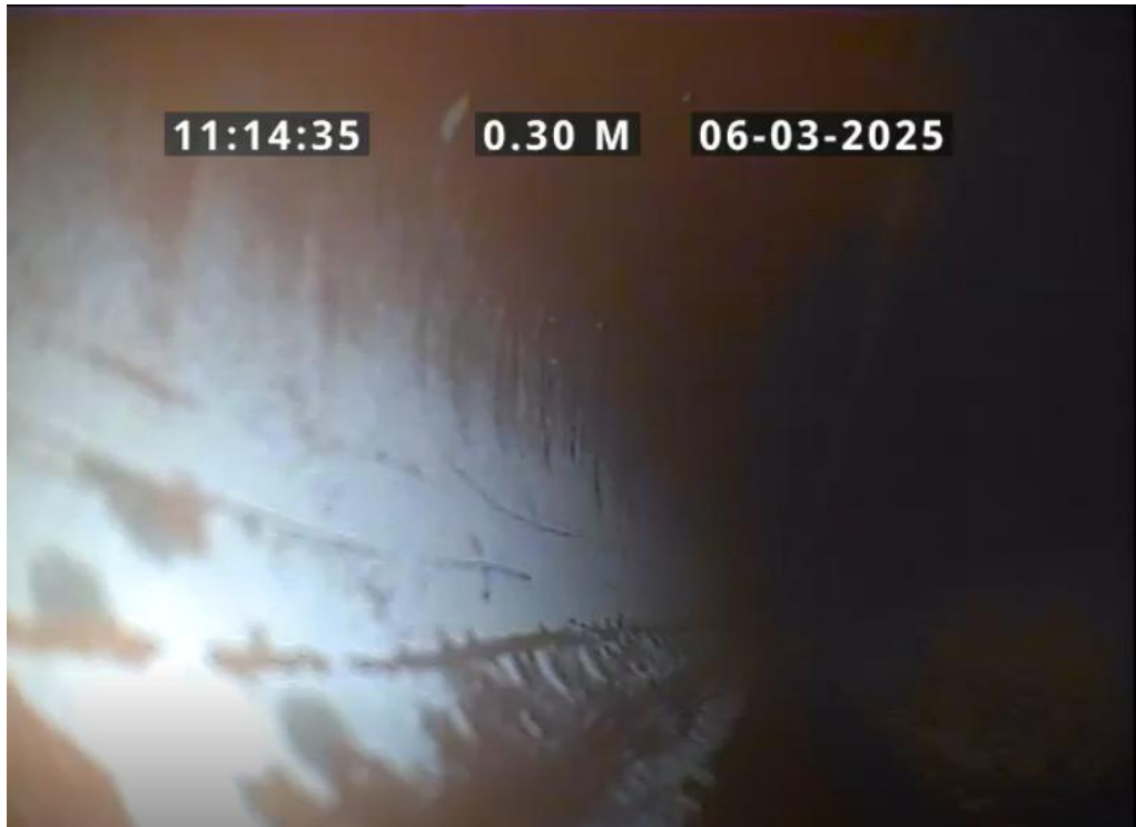
Start node, manhole, reference: PS251
