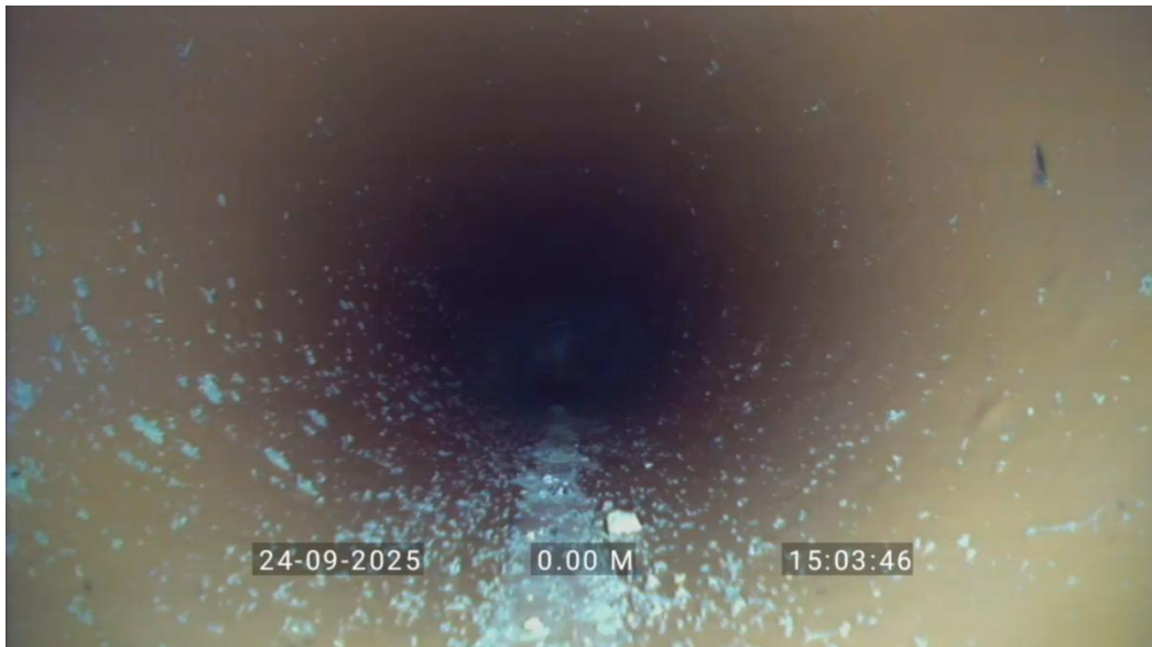
Start node, manhole, reference: PS220
