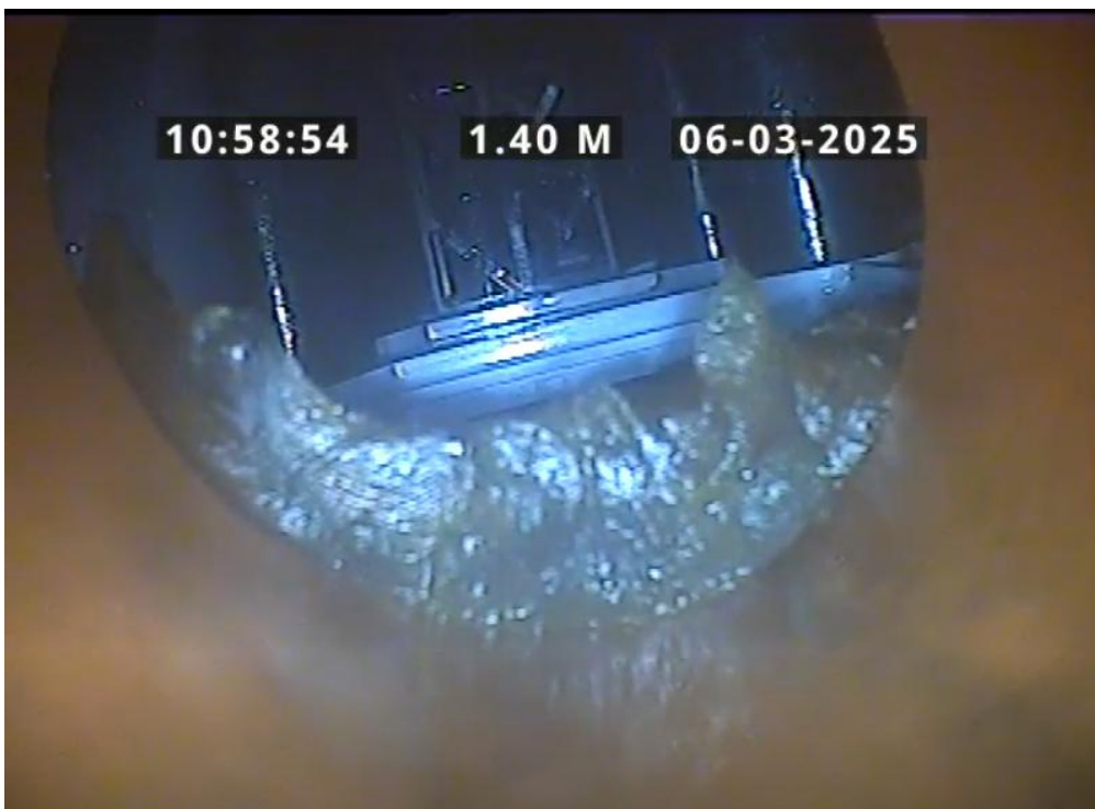
Finish node, soakaway, reference: SA66-67
