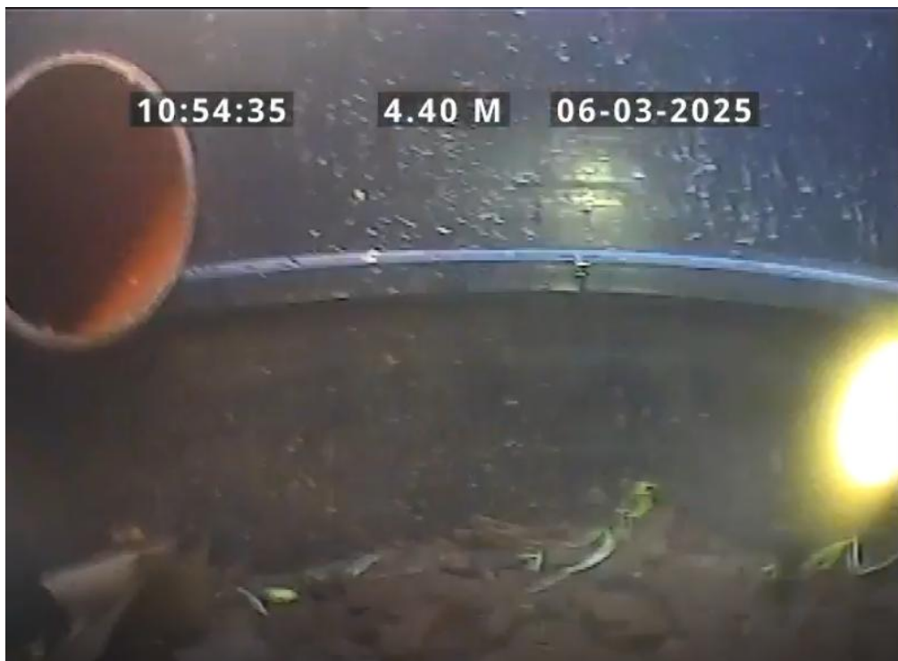
Finish node, manhole, reference: PSCP210
