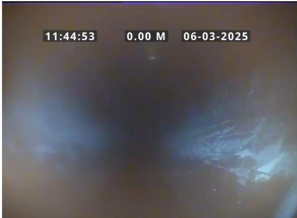
Start node, manhole, reference: PS221
