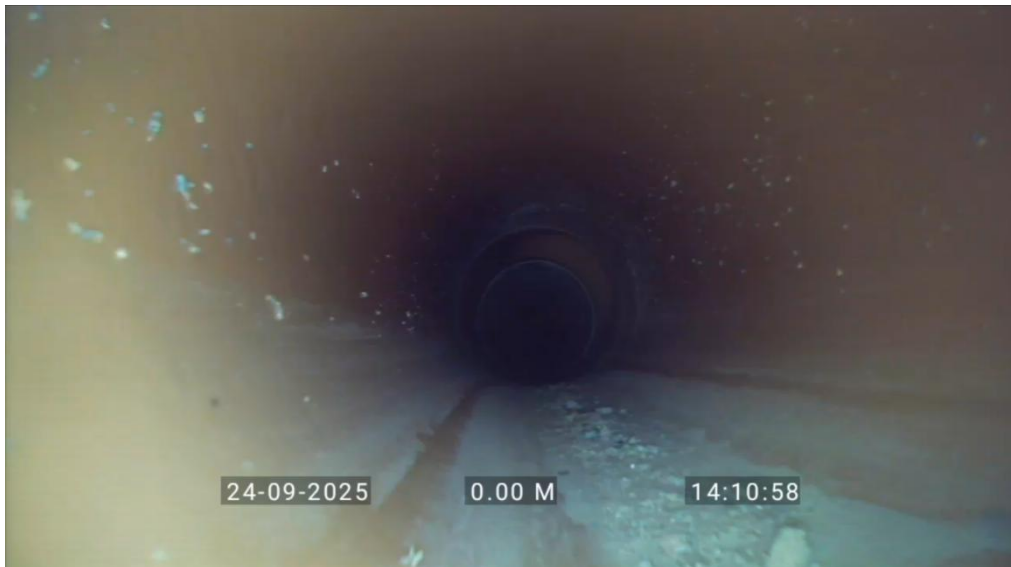
Start node, manhole, reference: PS54
