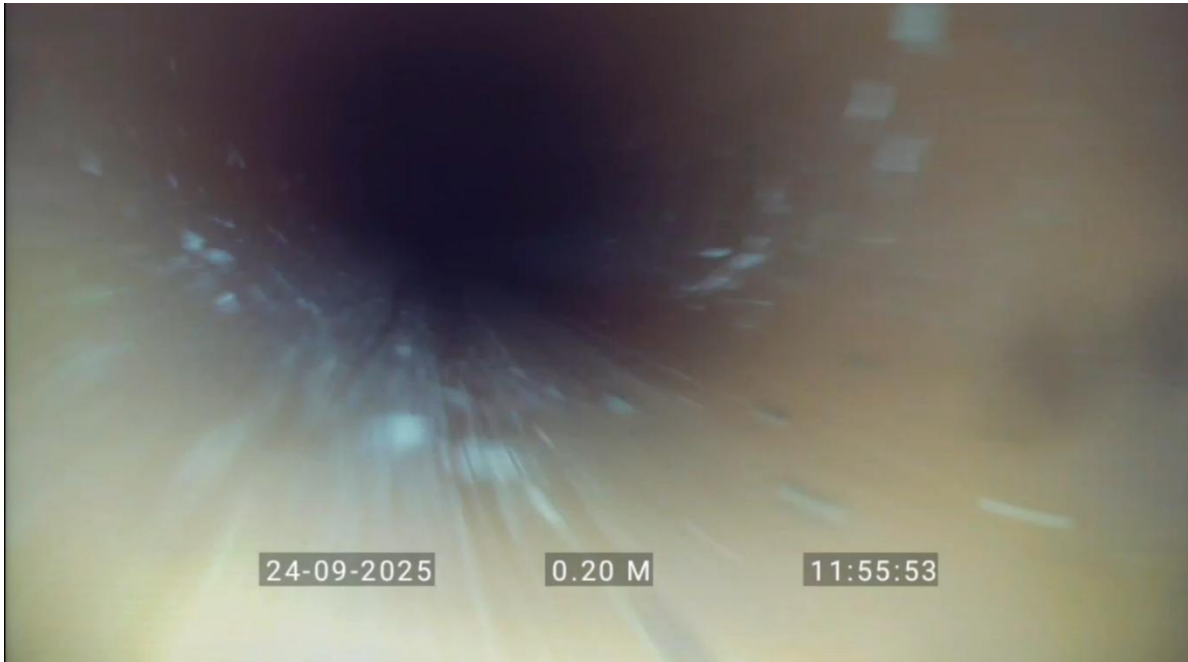
Start node, manhole, reference: PS5281
