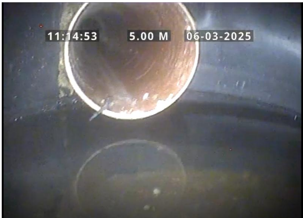
Finish node, manhole, reference: PSCP206
