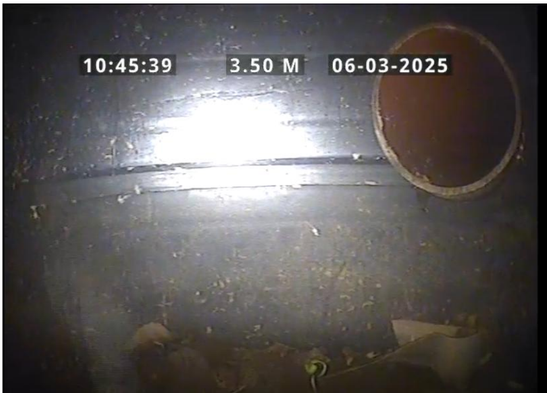
Finish node, manhole, reference: PSCP217
