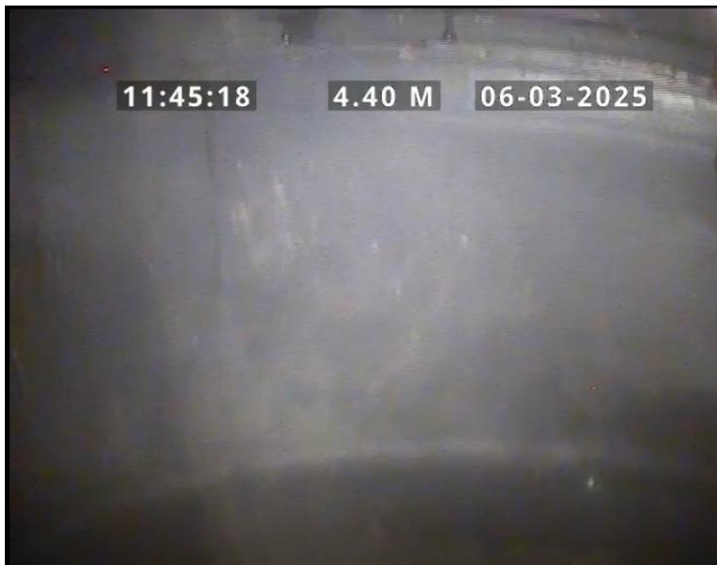
Finish node, manhole, reference: PSCP220
