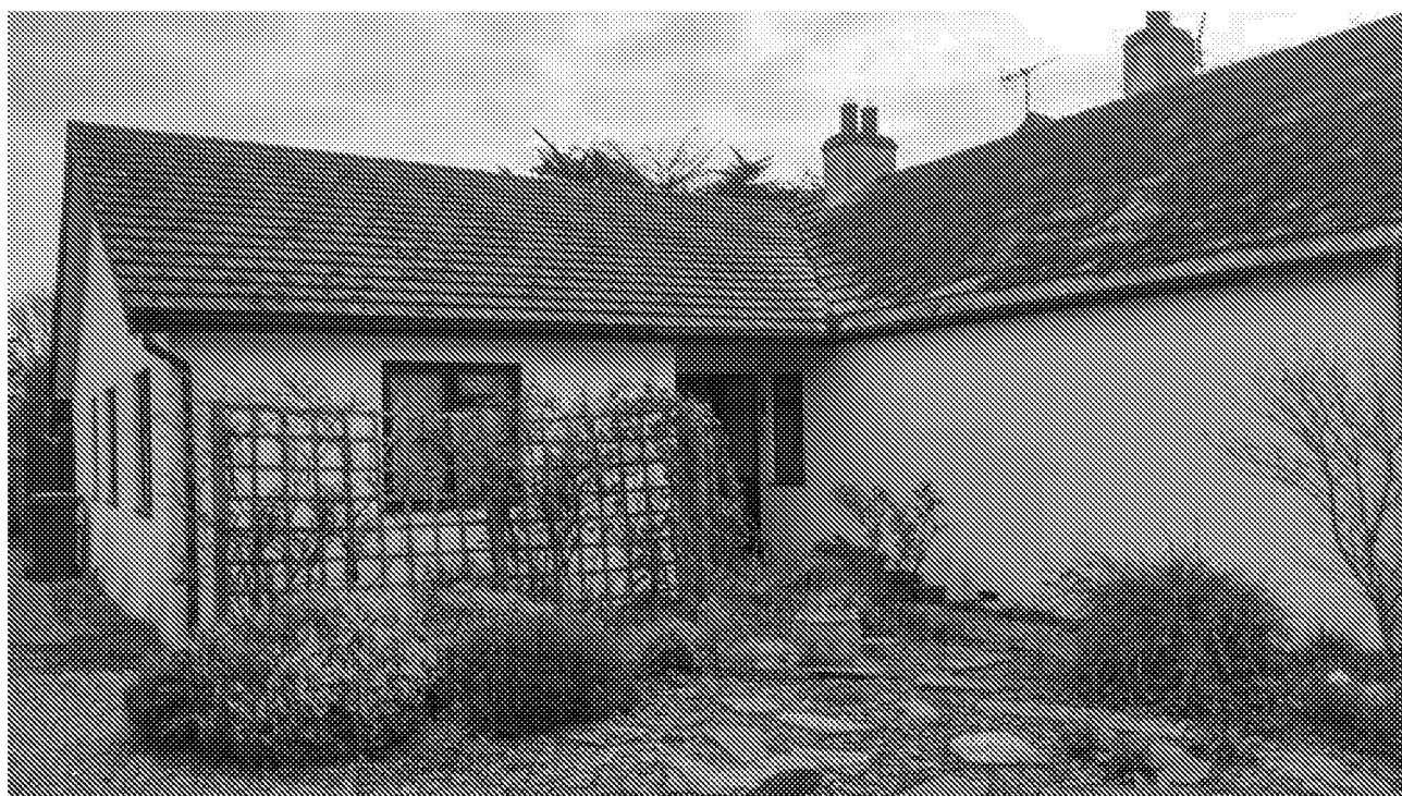
Photograph No. 1 - View of the dwelling from the entrance.
