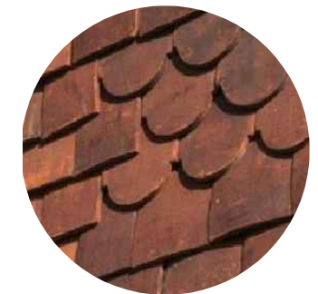
Upper Walls - Tile hanging
