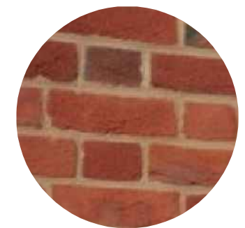
Lower Walls - Brick
