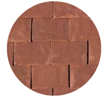
Roof - Clay tile
