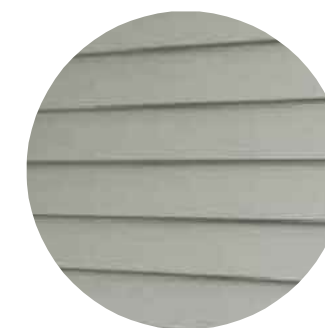
Upper Walls - Weatherboarding
