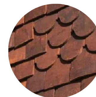
Upper Walls - Tile hanging
