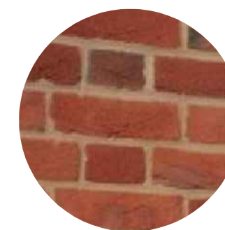
Lower Walls - Brick
